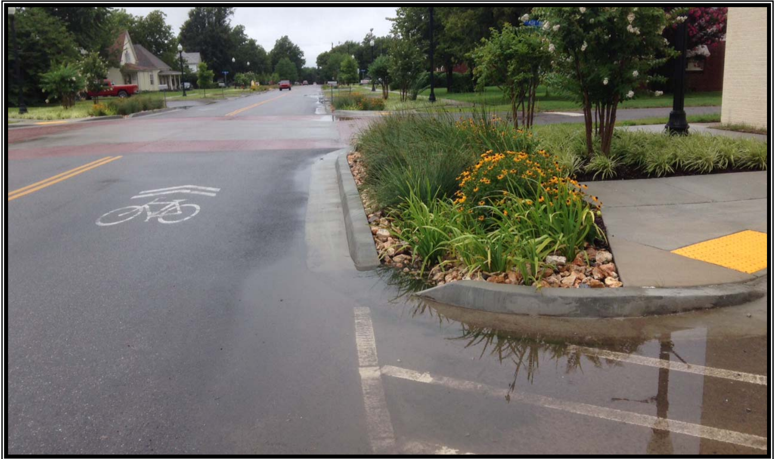
ONE OF THE RAIN GARDEN IMPROVEMENTS | ON BROADWAY, WEST OF MAIN STREET
