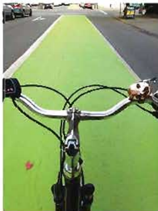
COLORLED PAVEMENT WITHIN A BICYCLE LANE INCREASES THE VISIBILITY OF THE FACILITY, IDENTIFIES POTENTIAL AREAS OF CONFLICT, AND REINFORCES PRIORITY TO BICYCLISTS
