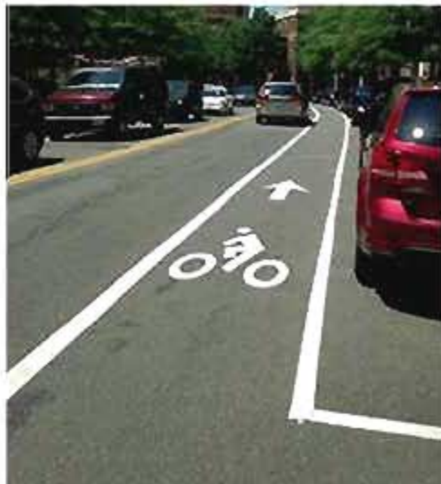
BIKE LANES ARE MARKED WITH A BICYCLIST SYMBOL AND ARROW INDICATING DIRECTION OF TRAVEL
