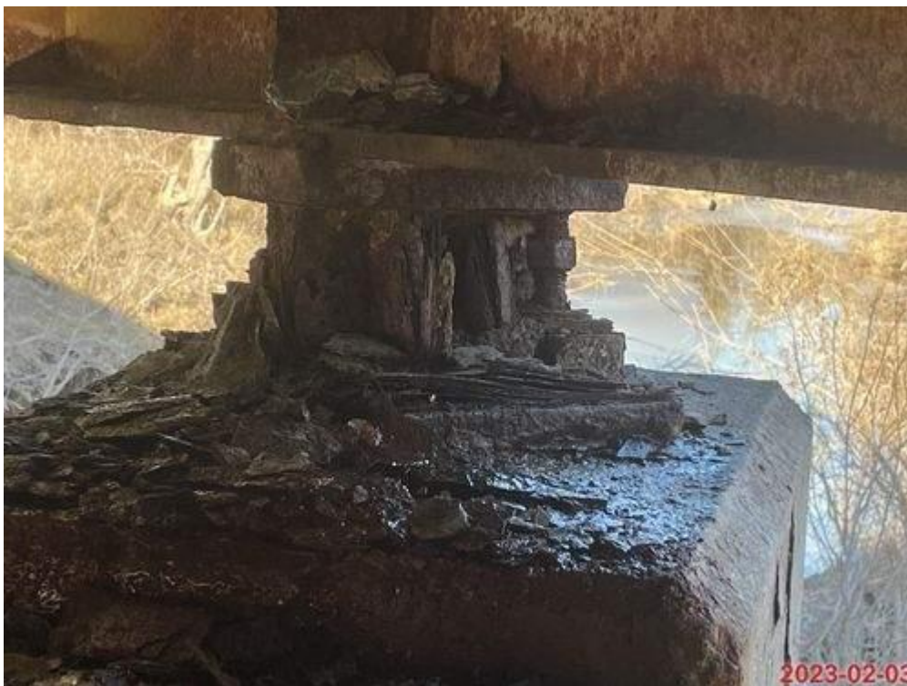
PHOTO 22: BEARING 4 AT PIER 1
