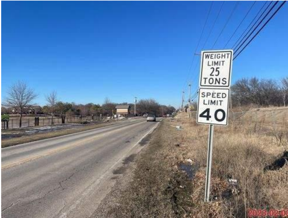
PHOTO 1: SOUTH APPROACH WITH 25 TON POSTING SIGNS (LOOKING NORTH)
