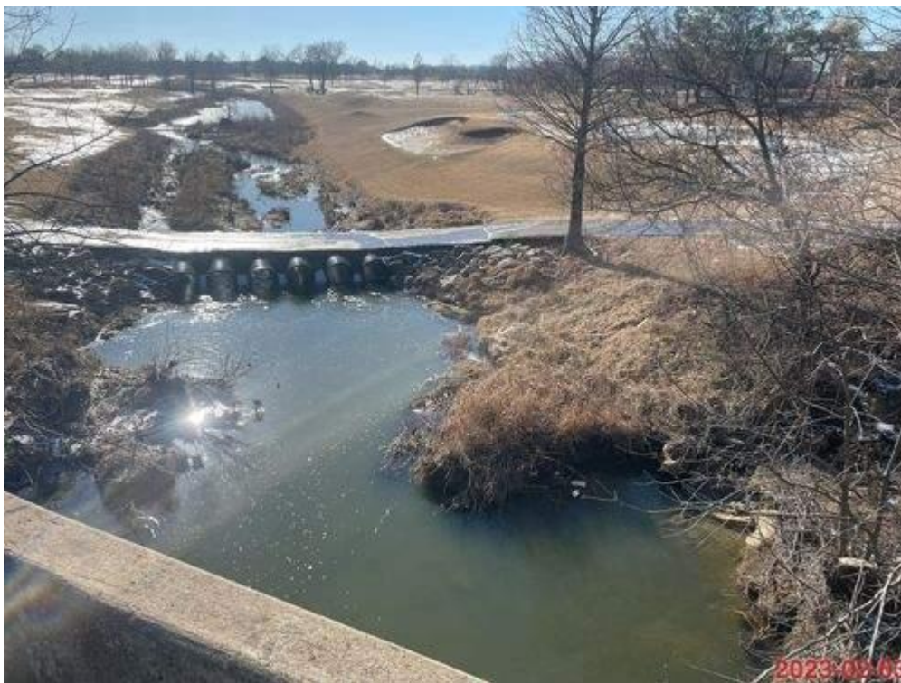
PHOTO 4: CHANNEL, UPSTREAM (LOOKING WEST)
