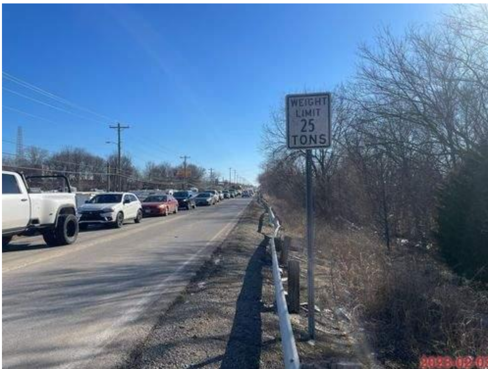
PHOTO 2: NORTH APPROACH WITH 25 TON POSTING SIGNS (LOOKING SOUTH)
