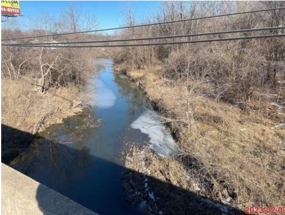
PHOTO 5: CHANNEL, DOWNSTREAM (LOOKING EAST)
