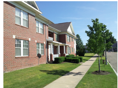
Figure 3.12 (top) and Figure 3.13 (bottom) Illustrates the Flats building form which increases density in single-family areas and provides an additional housing option in commercial and mixed-use areas.
