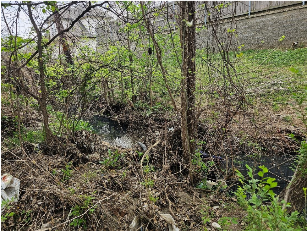
Section of Channel
