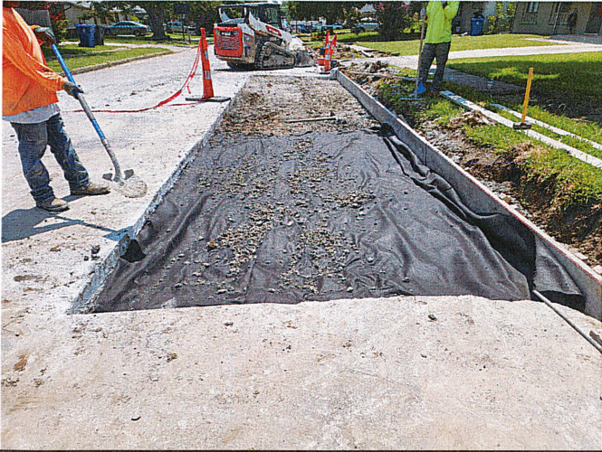
Fabric on top of dirt Hickory Avenue
