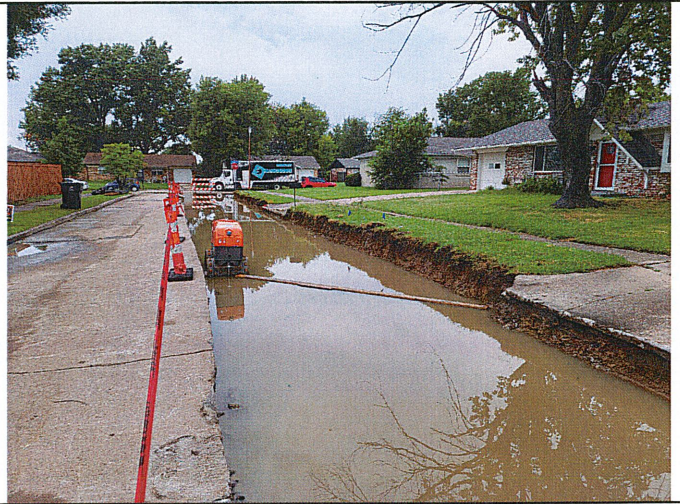
Subgrade holding 2' of water.
