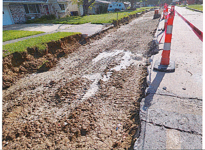
W. El Paso Pl. Dry solid subgrade. Holds up 4 ton skidloader. Dried up concrete washout.
