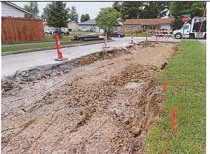
Hole to be filled in and subgrade cub to grade W. El Paso Pl
