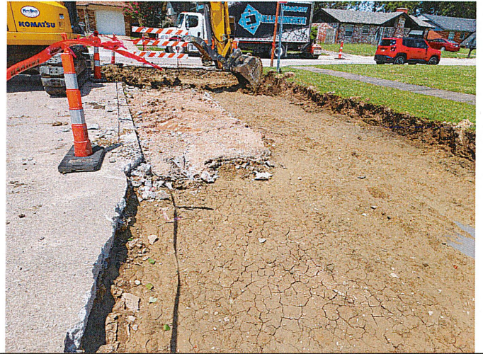
Subgrade from panel that did not have to be removed El Paso Place
