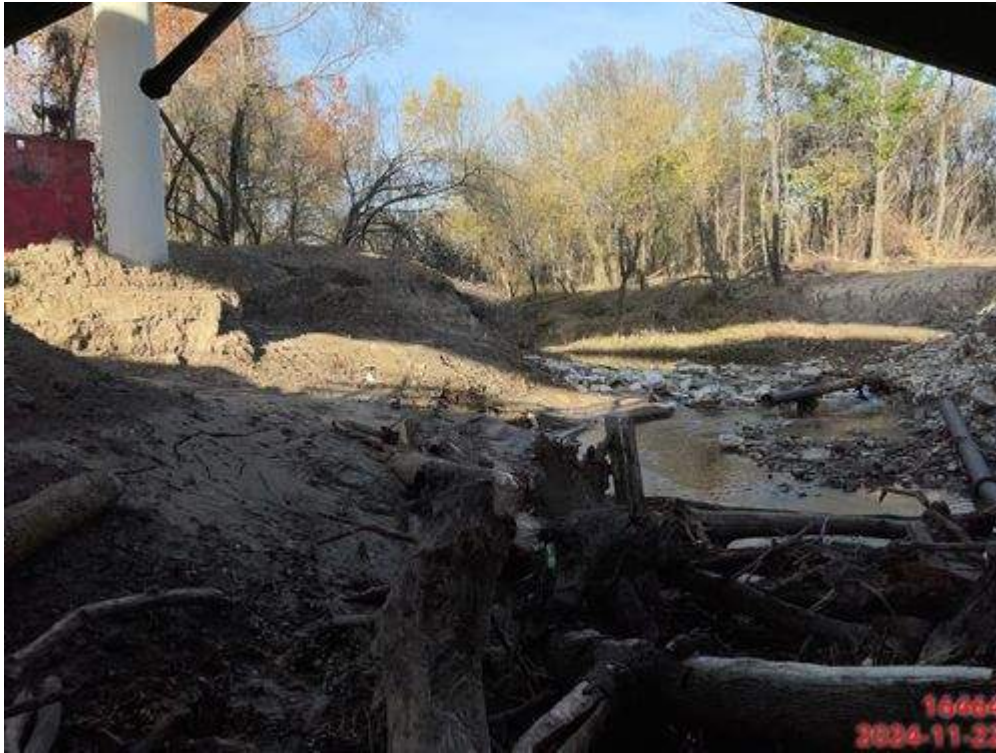
PHOTO 3: CHANNEL, UPSTREAM (LOOKING NORTH)
