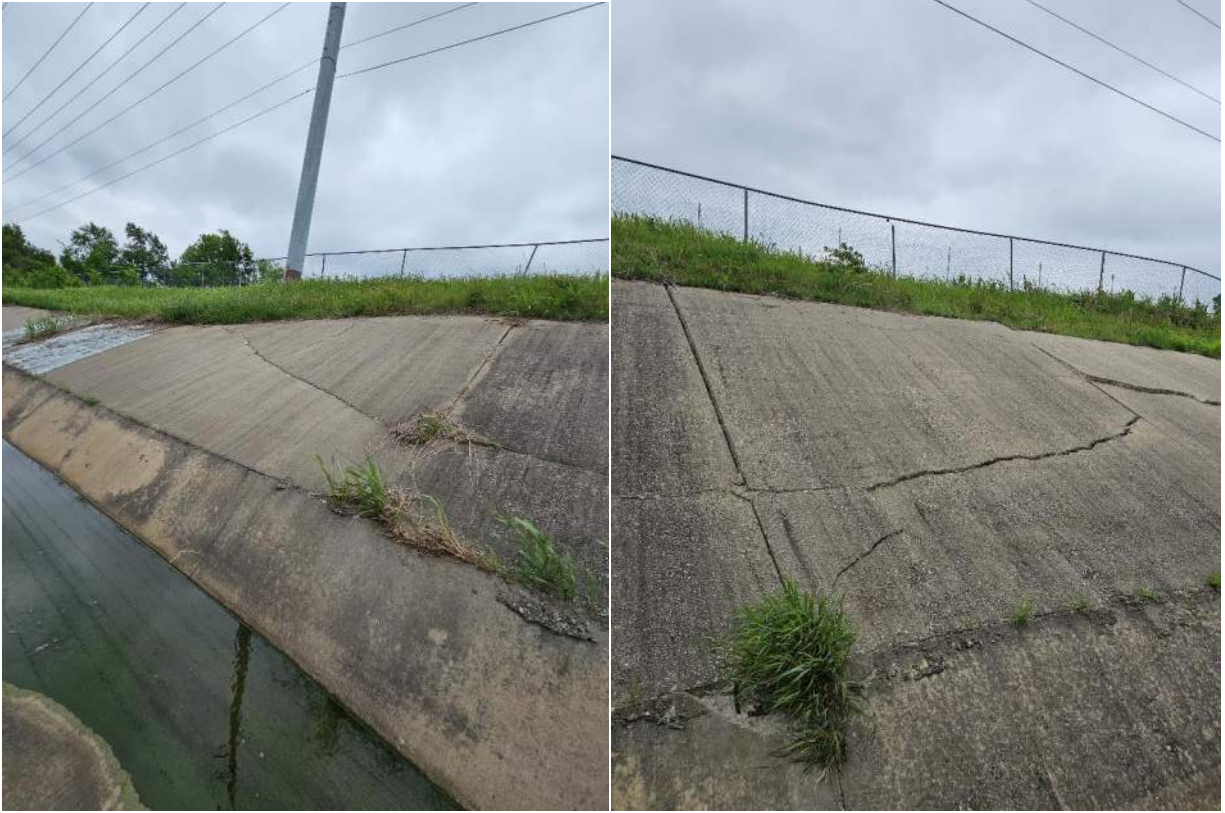
Cracks along the West wall of channel
