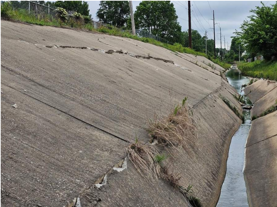
Flow line of channel reduced
