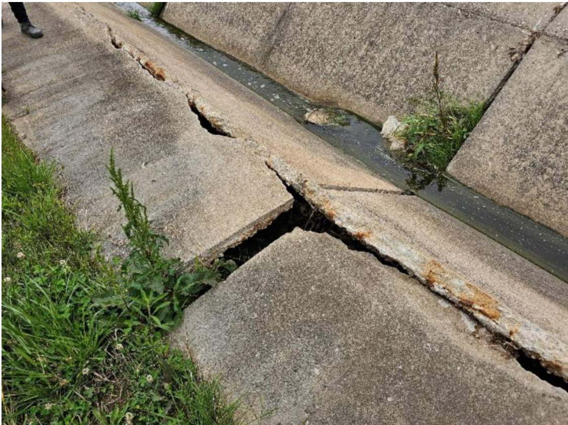
West side of channel buckle, East side of channel appears to have slid
