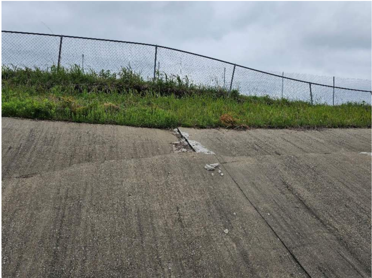
Cracks along the West wall of channel
