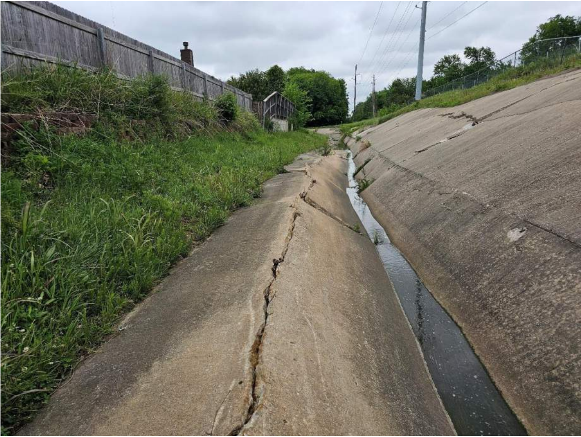
West side of channel buckle, East side of channel appears to have slid
