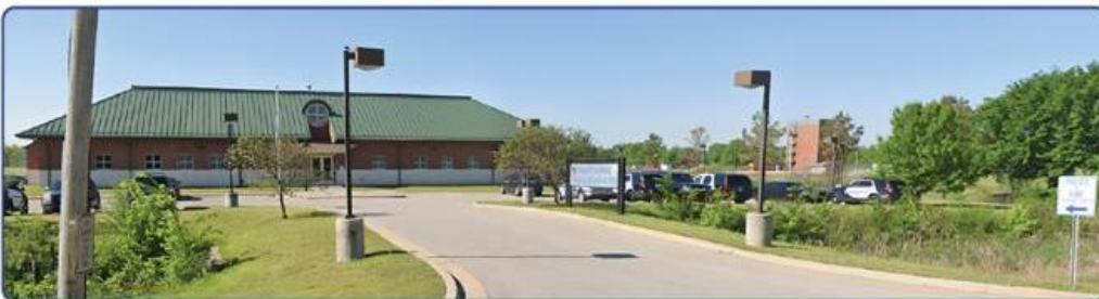
EXISTING CAMPUS ENTRANCE
