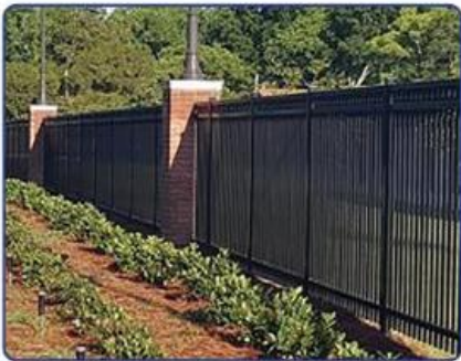
FENCE WITH MASONRY COLUMNS EXAMPLE
