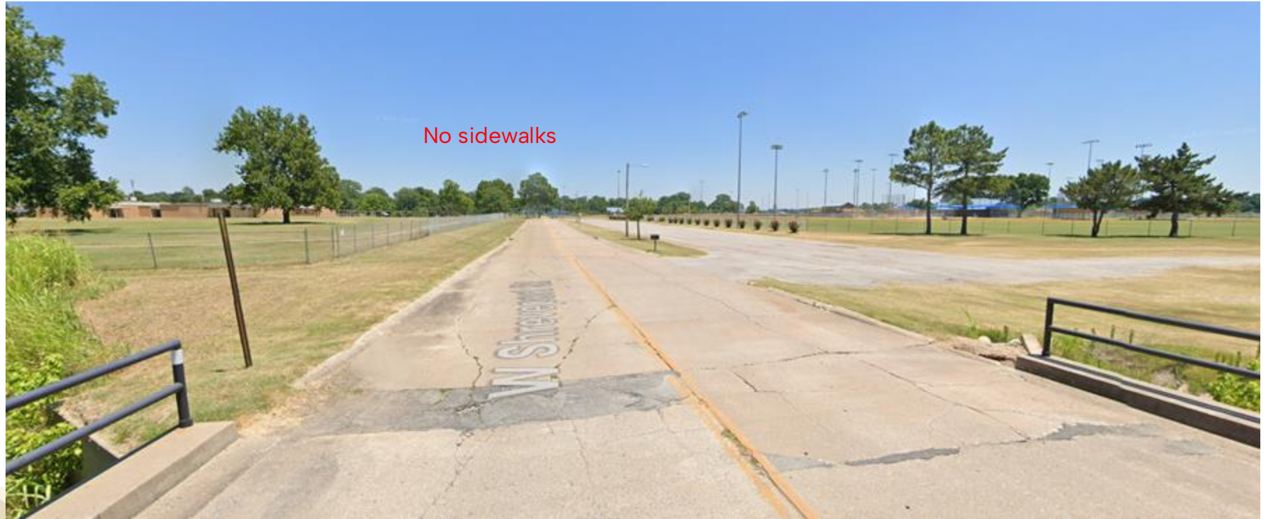
Looking East from Bridge on Shreveport Street June 2022
