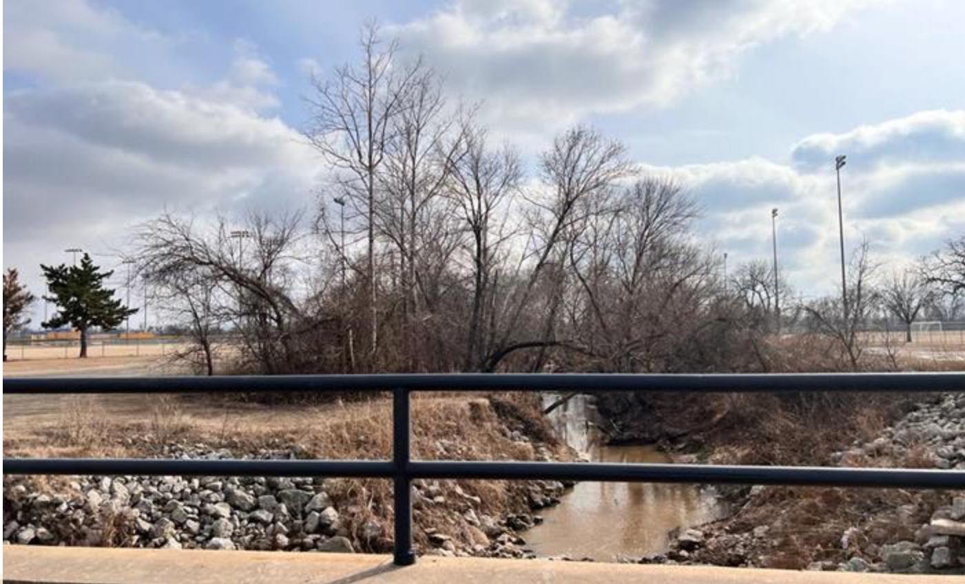
Looking North from Bridge on Shreveport Street
