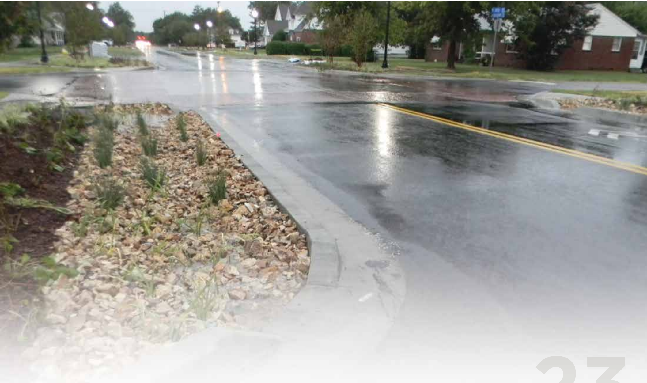
The rain gardens on Broadway Avenue enhance the landscape and prevent flooding.
