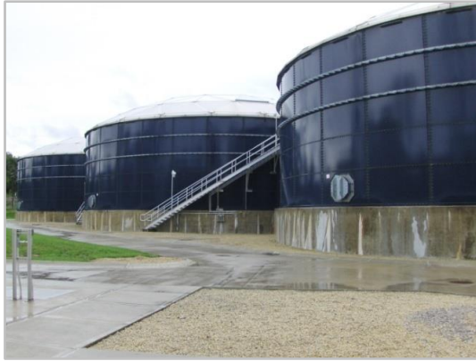
Cincinnati MSD Three 1.2 MG Tanks Exterior Finishes can be Customized
