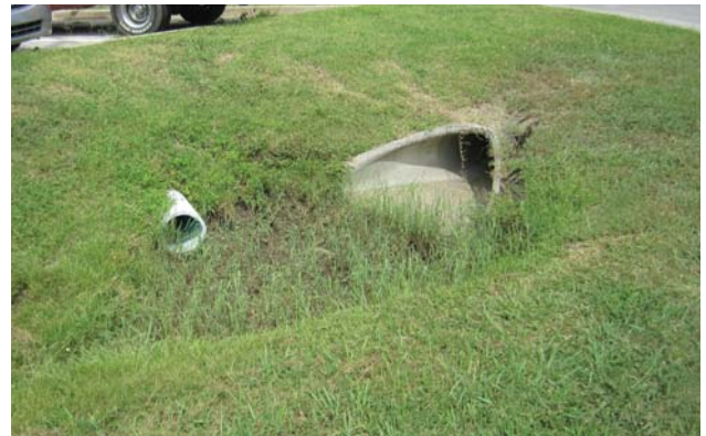
Drain pipe at Municipal Court north driveway - Looking west
