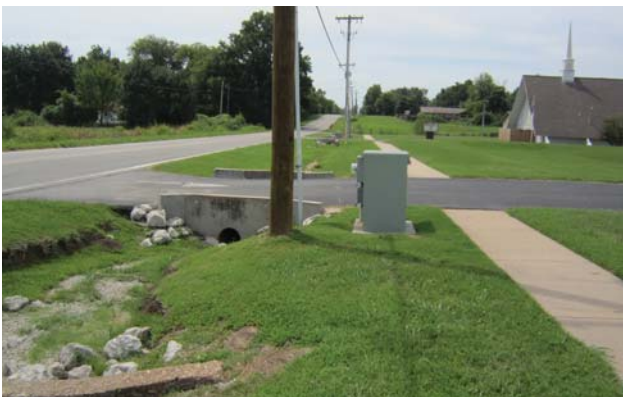
Faith Baptist Church existing utilities at center driveway- Looking south
