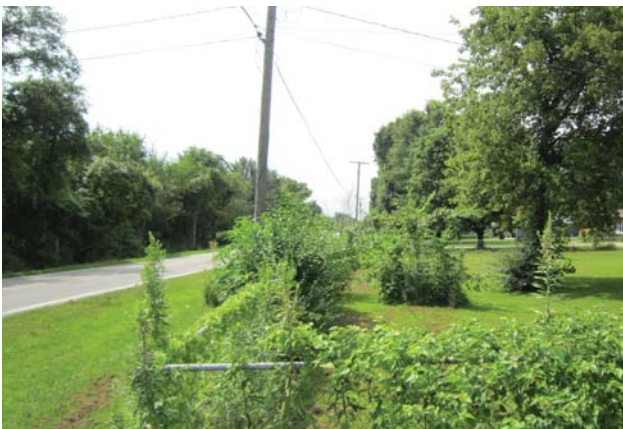
1st Pl. fence encroachment - Looking south
