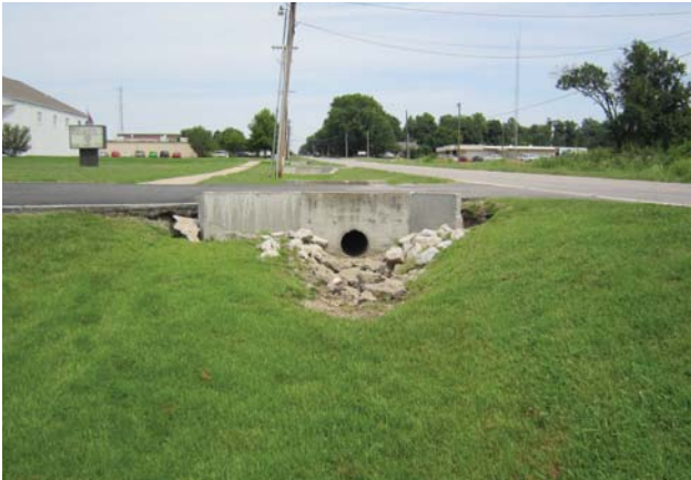
Faith Baptist Church south driveway - Looking north
