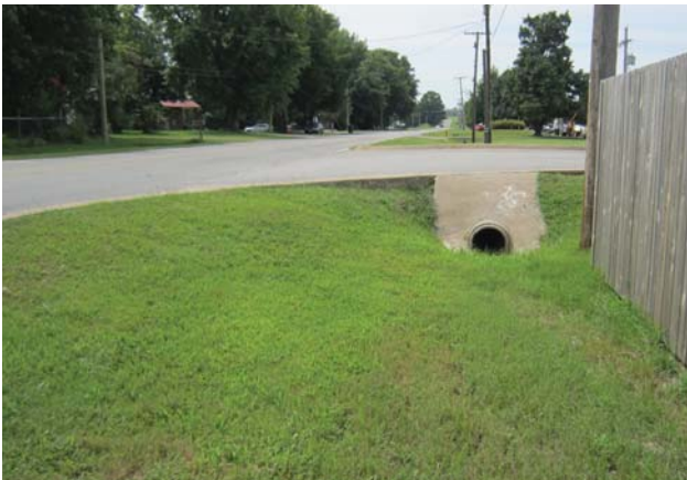
Police Station north driveway- Looking south
