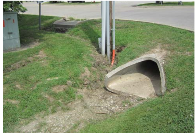
Drainage structures at Municipal Court south driveway - Looking north west
