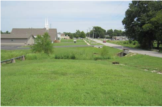
North side of Ithica Pl. - Looking north
