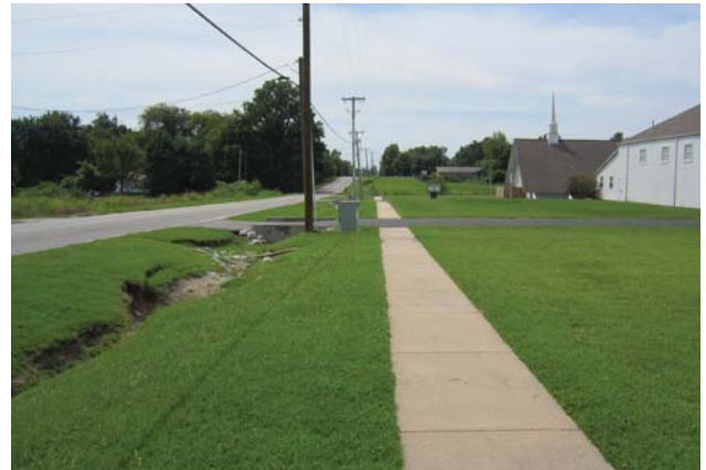
Faith Baptist Church existing sidewalk at center driveway - looking south
