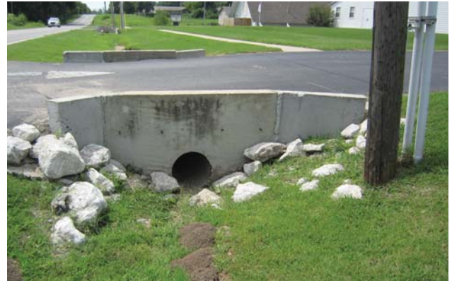
Faith Baptist Church center driveway - looking south
