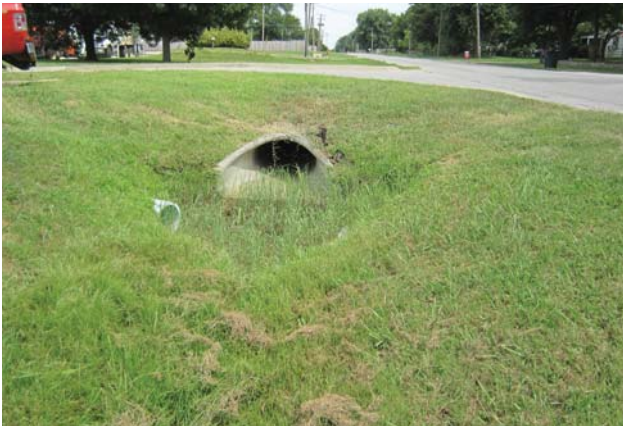
Municipal Court north driveway- Looking north
