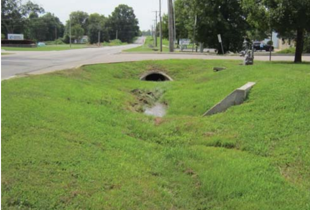
Municipal Court south driveway - looking south
