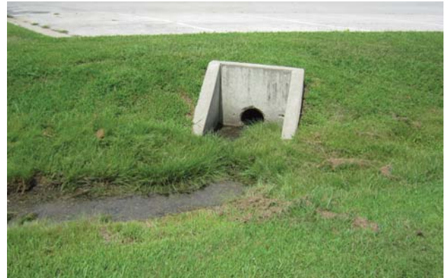
Drainage structure at Municipal Court south driveway - Looking west
