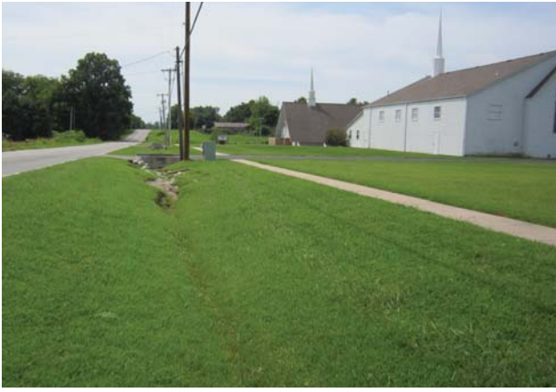
Faith Baptist Church - Looking south
