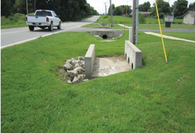
Faith Baptist Church drainage structure at south driveway - looking south
