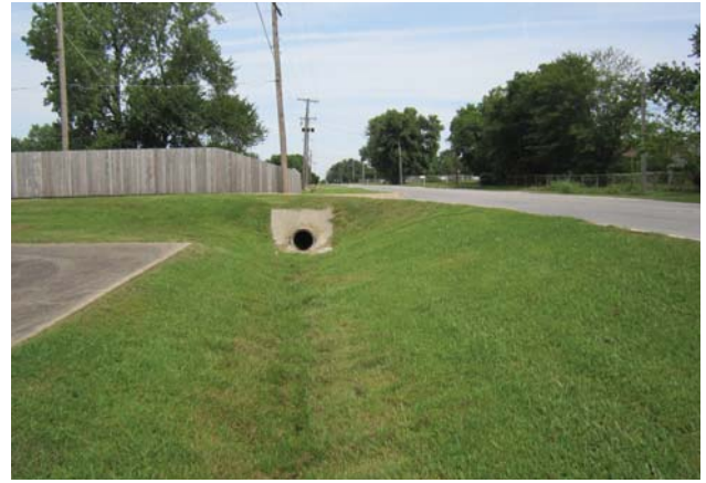
Police Station north driveway- Looking north
