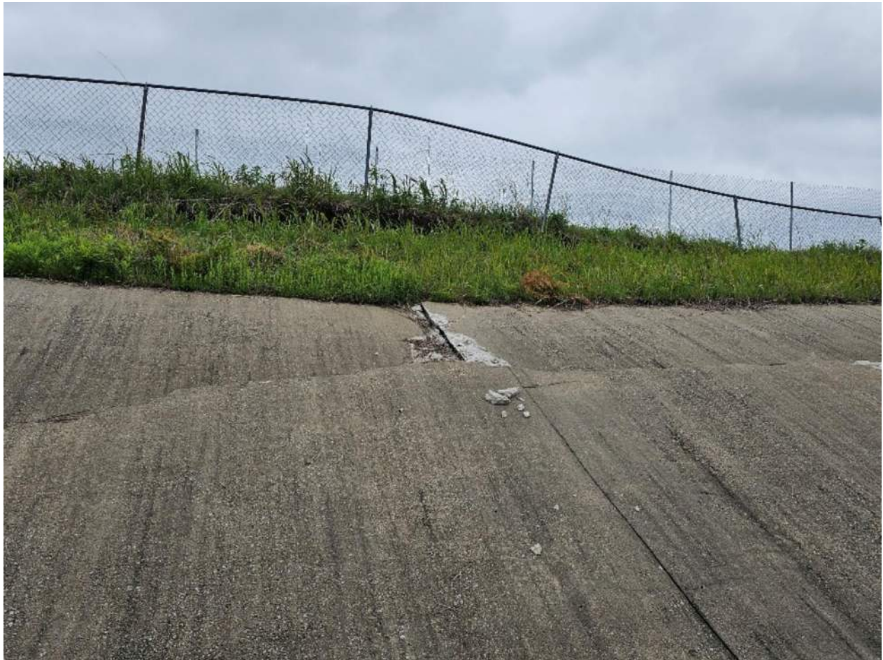
Cracks along the West wall of channel
