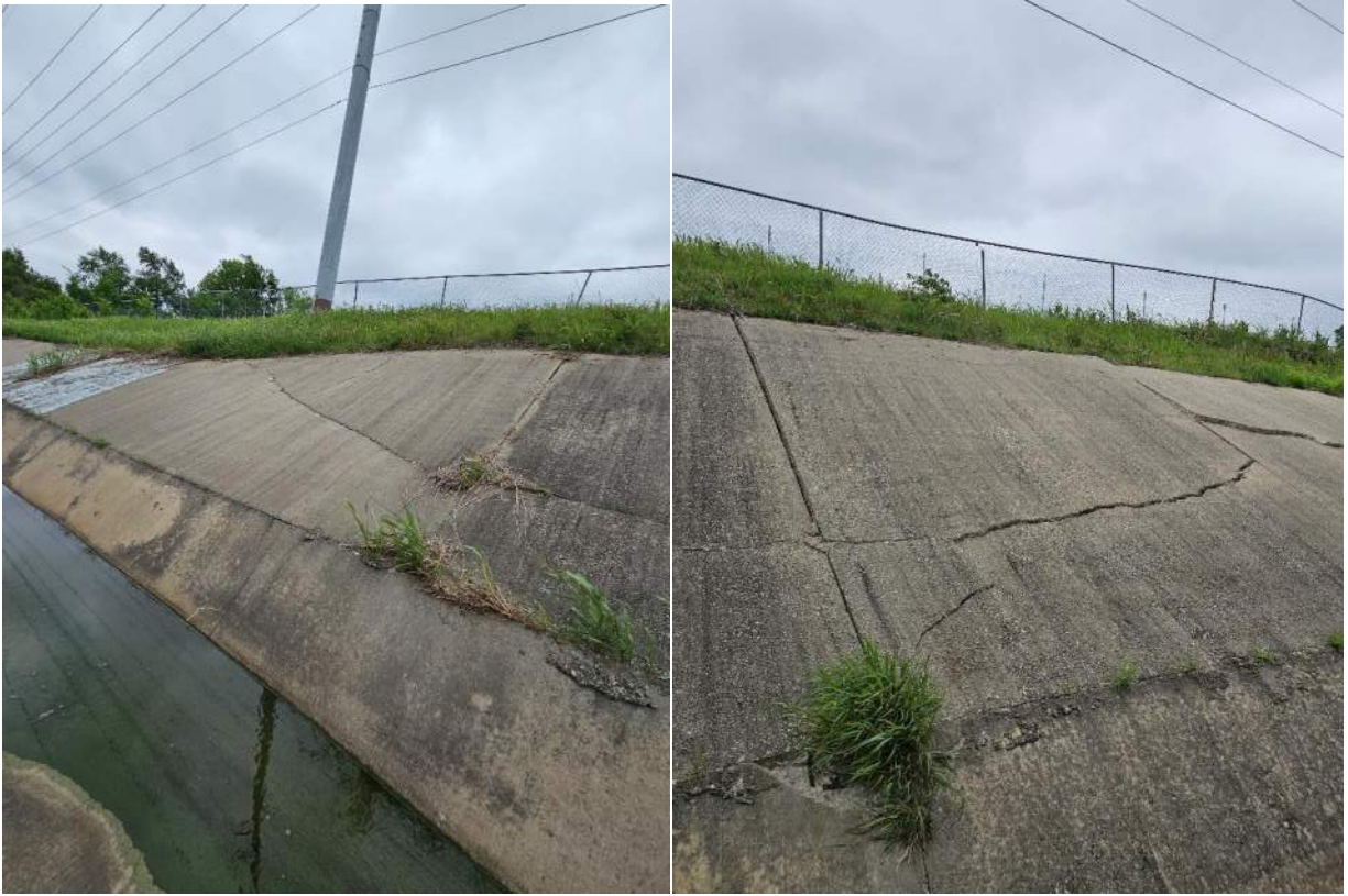
Cracks along the West wall of channel
