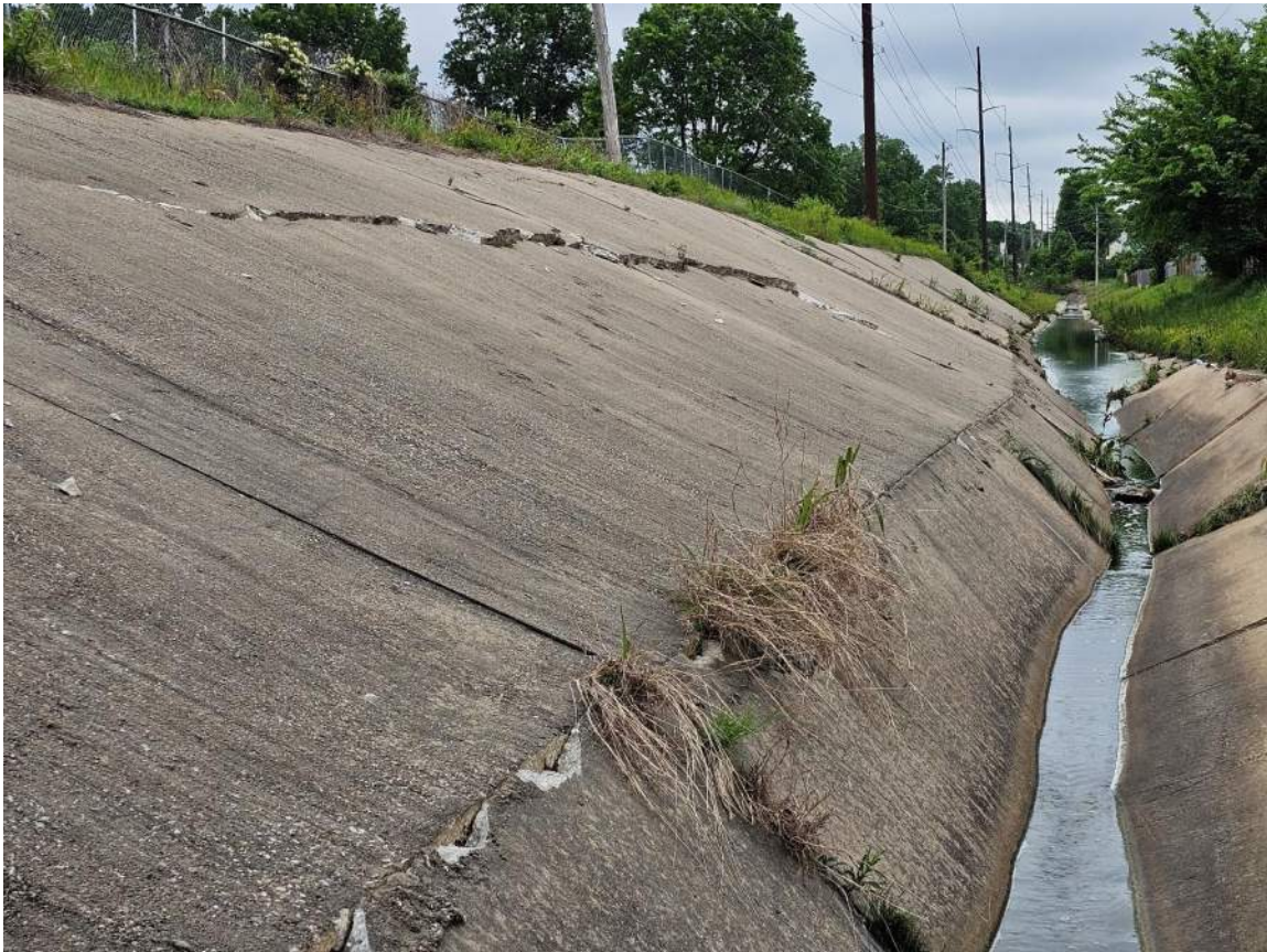
Flow line of channel reduced
