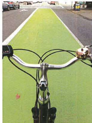
COLOR PAVEMENT WITHIN A BICYCLE LANE INCREASES THE VISIBILITY OF THE FACILITY, IDENTIFIES POTENTIAL AREAS OF CONFLICT, AND REINFORCES PRIORITY TO BICYCLISTS
