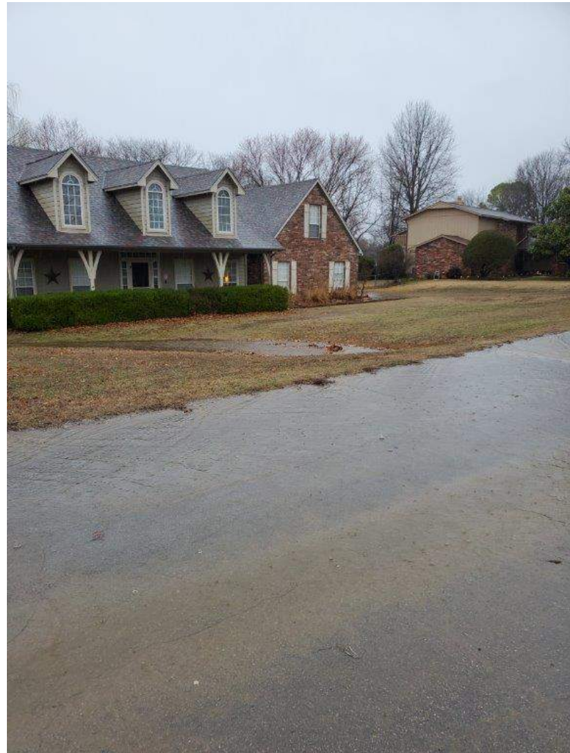
West side of S. Harp Blvd. – Existing Cross Drain
