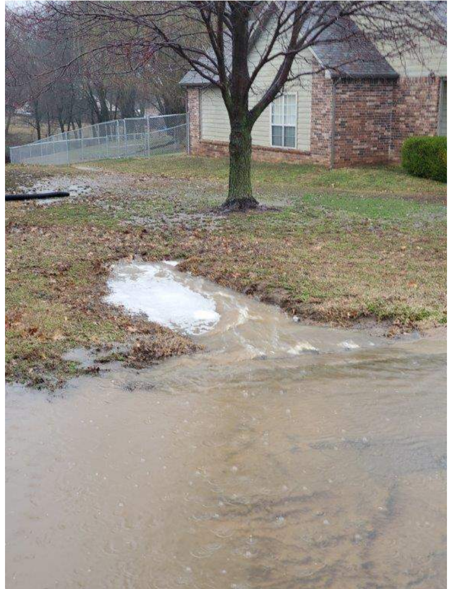
Small Drain on the applicant's property is overwhelmed
