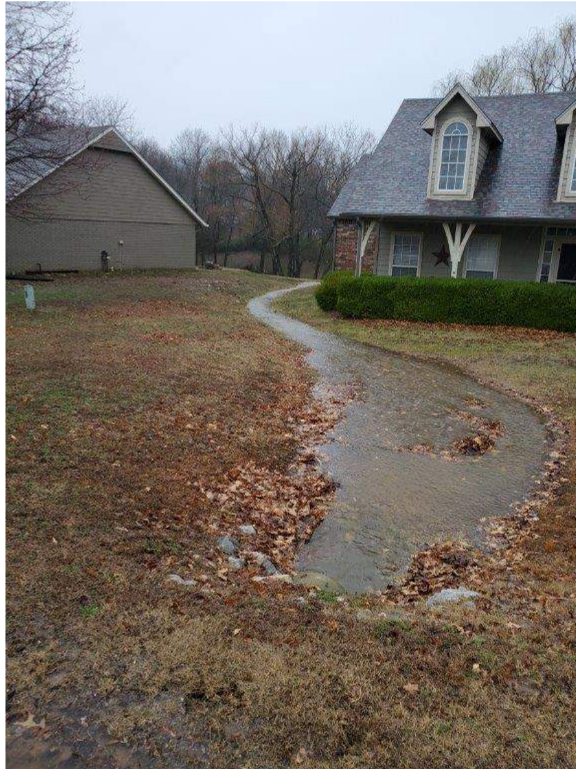
Neighbor to the north of applicant – cross drain swale
