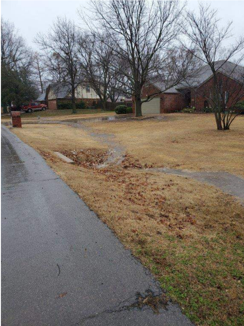
East side of S. Harp Blvd. – Existing Cross Drain
