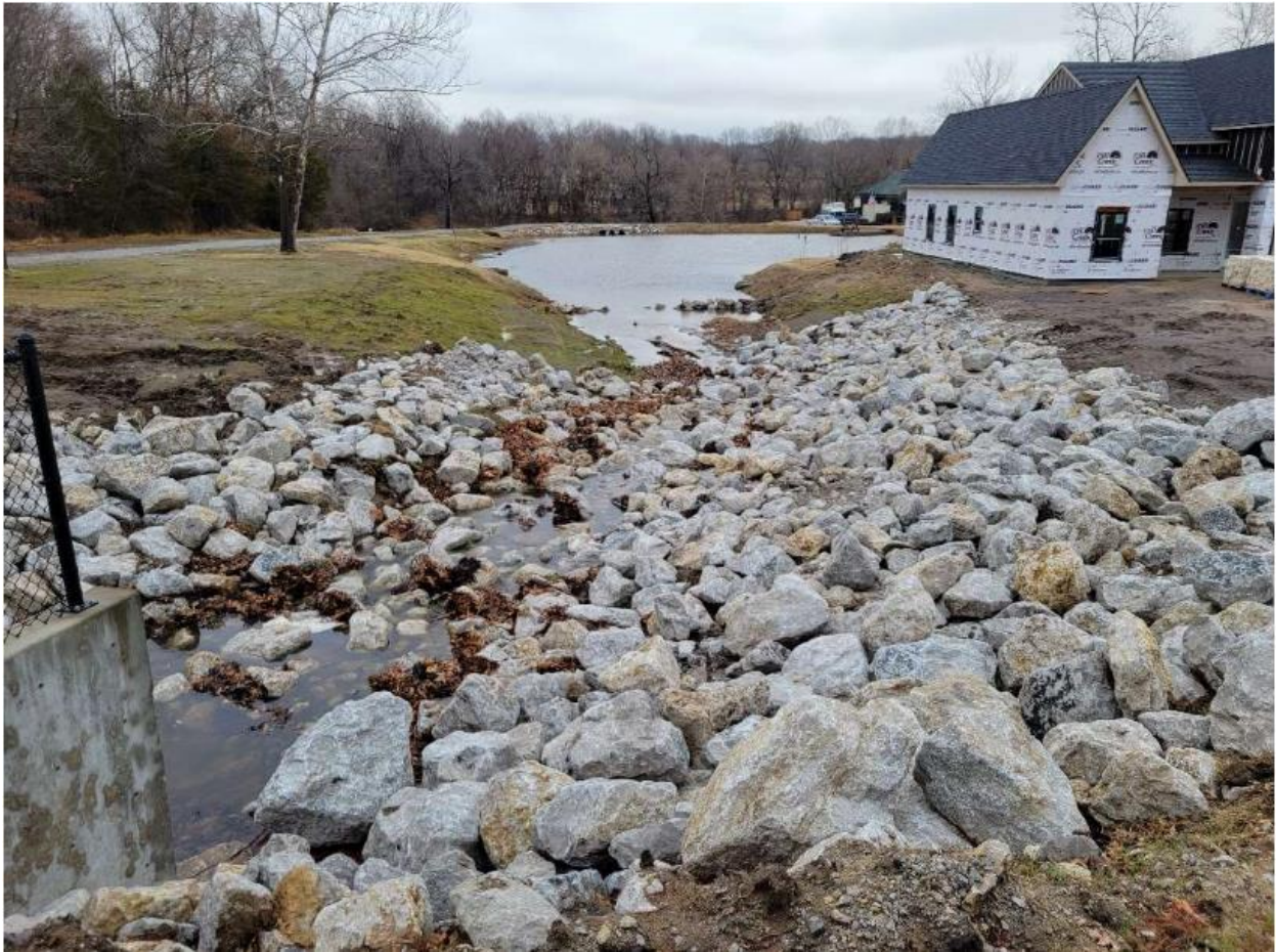
Picture 6: Standing at Lynn Lane looking east towards Broken Arrow Creek. Previous DAC improvements from Case Number 20-003 Agenda Item 20-1193. Improvements complete in 2021. Total amount spent was $76,131.66 for upsizing culvert and addressing erosion from culvert.
