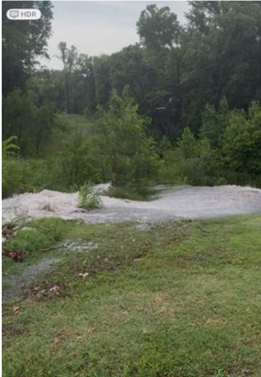
Picture 1: Overflow Weir Channel from Private Pond looking upstream Broken Arrow Creek
