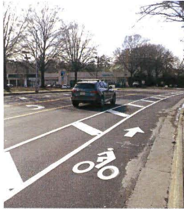
BUFFERED BIKE LANES PROVIDE GREATER SHY DISTANCE BETWEEN MOTOR VEHICLES AND BICYCLISTS
