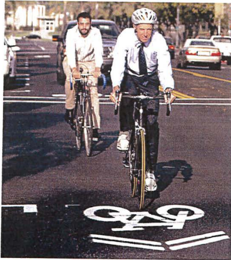
Shared lane markings indicate bicyclists' presence to drivers and appropriate placement on the roadway
