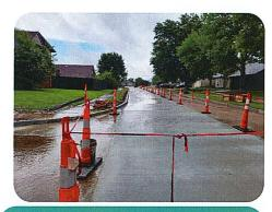
We need to make sure we are establishing a crown in the road and directing the water to the outters.
