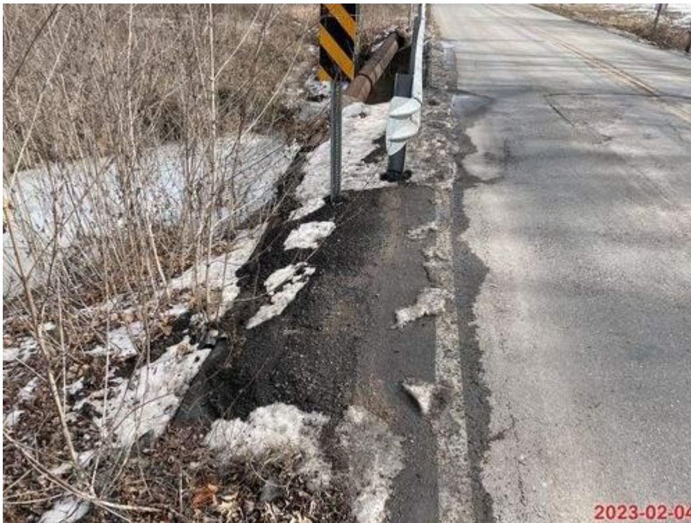
PHOTO 10: MINOR EROSION AT NW CORNER REPAIRED
