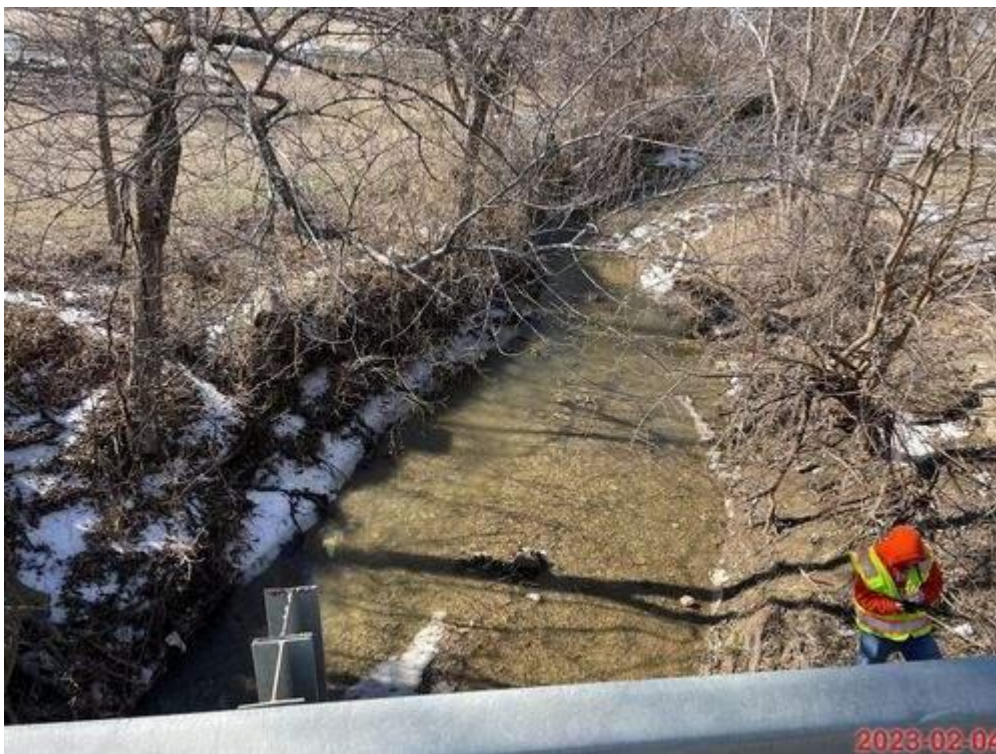
PHOTO 4: CHANNEL, UPSTREAM (LOOKING WEST)
