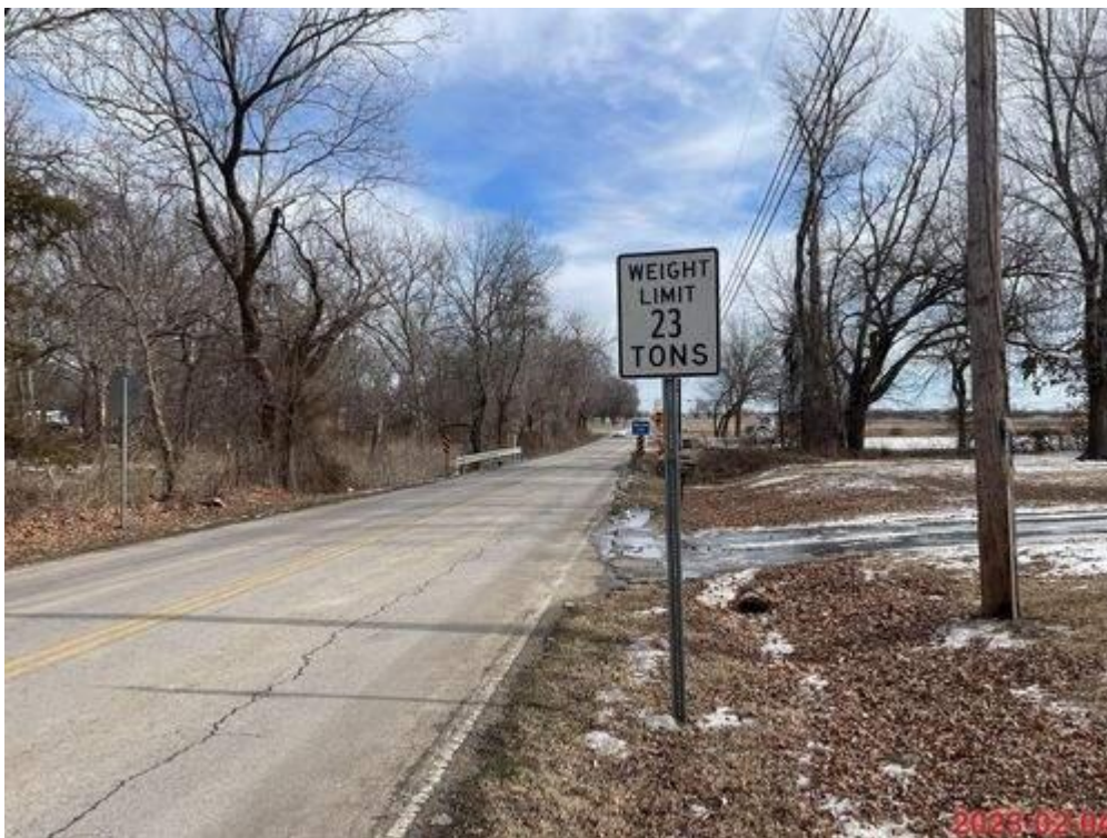
PHOTO 2: WEST APPROACH WITH 23 TON POSTING SIGN (LOOKING EAST)
