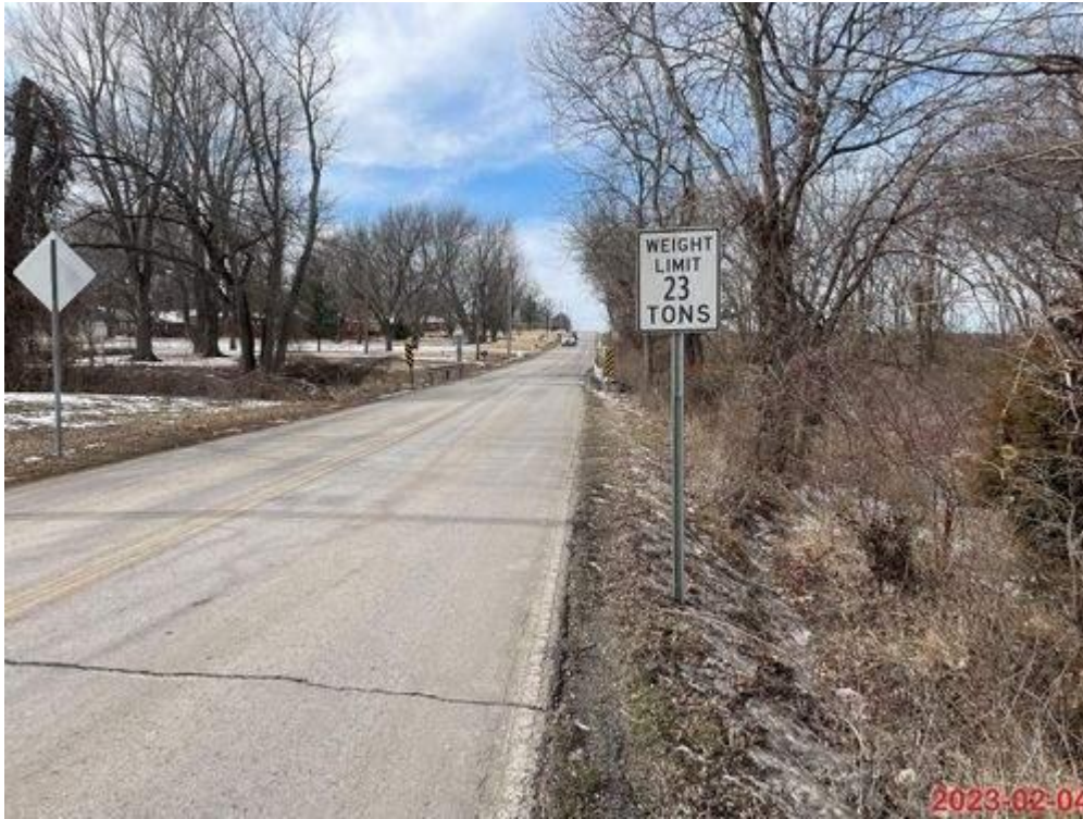
PHOTO 1: EAST APPROACH WITH 23 TON POSTING SIGN (LOOKING WEST)
