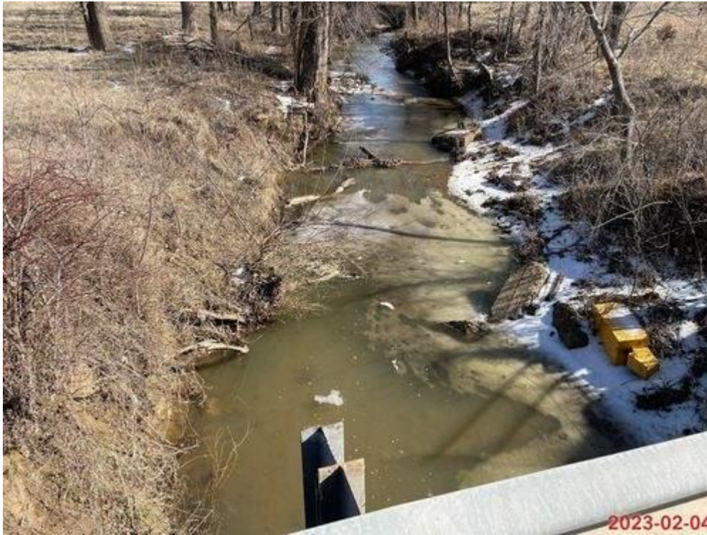
PHOTO 5: CHANNEL, DOWNSTREAM (LOOKING EAST)
