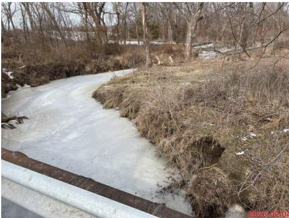
PHOTO 4: CHANNEL, UPSTREAM (LOOKING NORTH)
