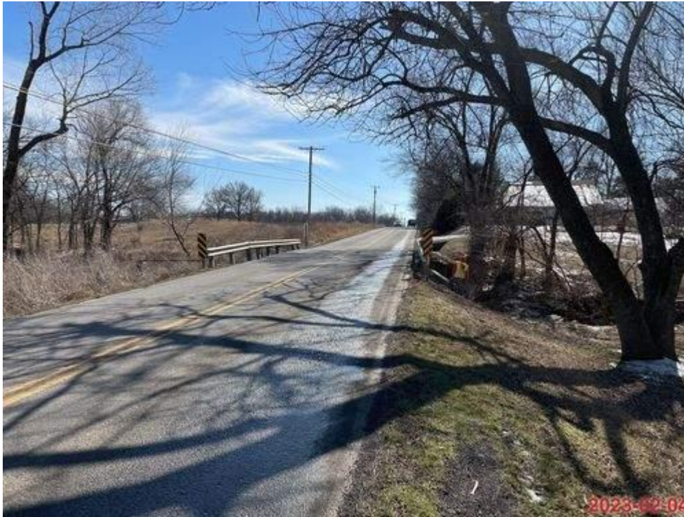
PHOTO 1: NORTH APPROACH (LOOKING SOUTH)
