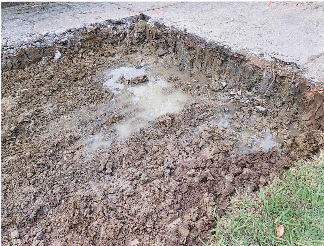
Figure 20: Material wet, chipping, bent rebar, no sawcut
