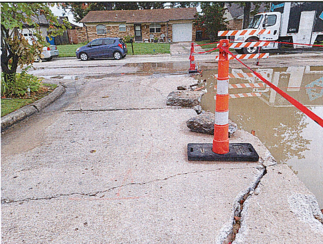
Subgrade holding 2' of water at S. Hickory Pl. and W. El Paso Pl.
