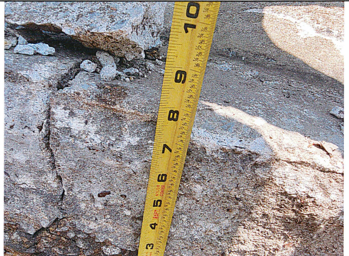
Existing concrete 7-3/4 inches thick El Paso Place
