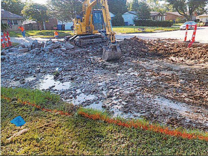
W. El Paso Pl. Dry solid subgrade. Holds up 4 ton skid loader.
