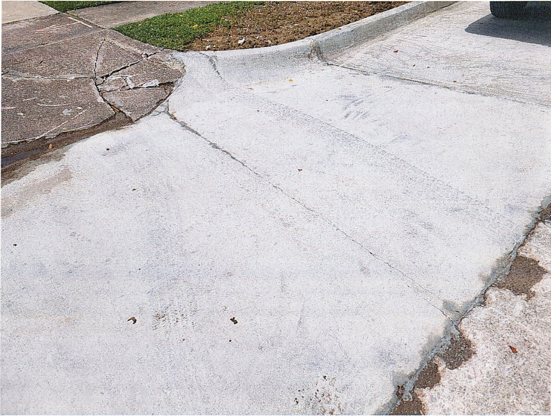
Figure 23: Structural Crack due to improper methods
