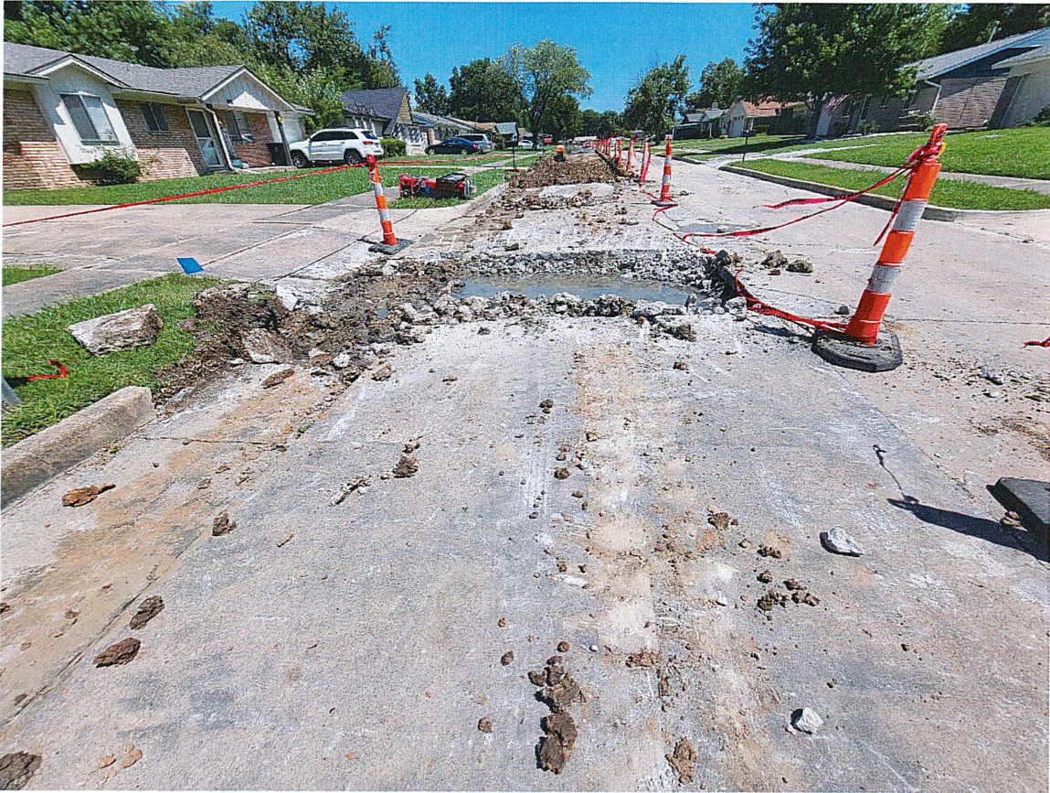
Figure 5: Teeth marks showing excavator used to break concrete
