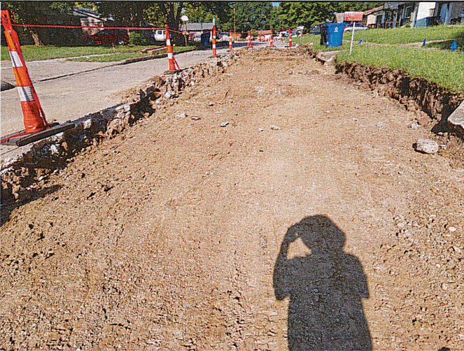
W. El Paso Pl. Dry solid subgrade. Holds up 4 ton skid loader.
