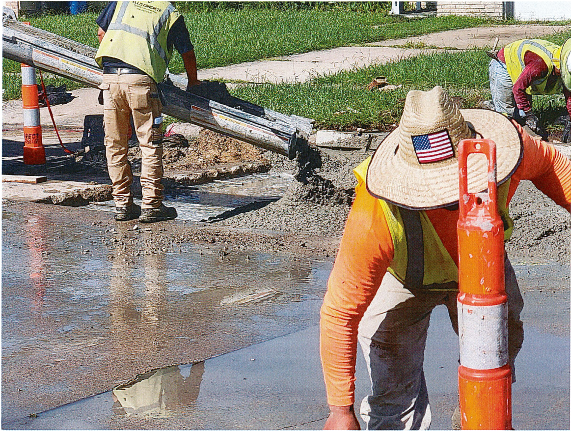
Figure 15: Not pumping out water, but still pouring with too much water in hole
