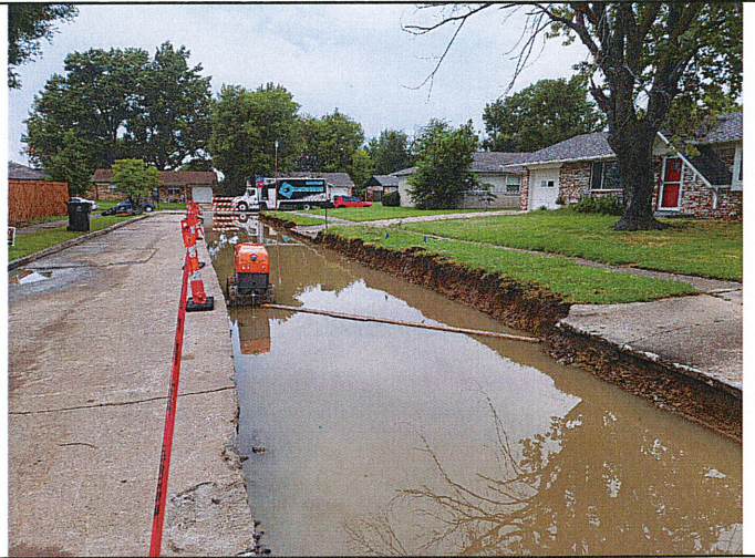
Subgrade holding 2' of water.
