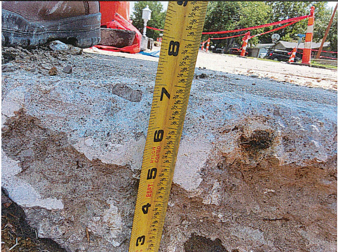
Existing concrete 7 inches thick El Paso Place
