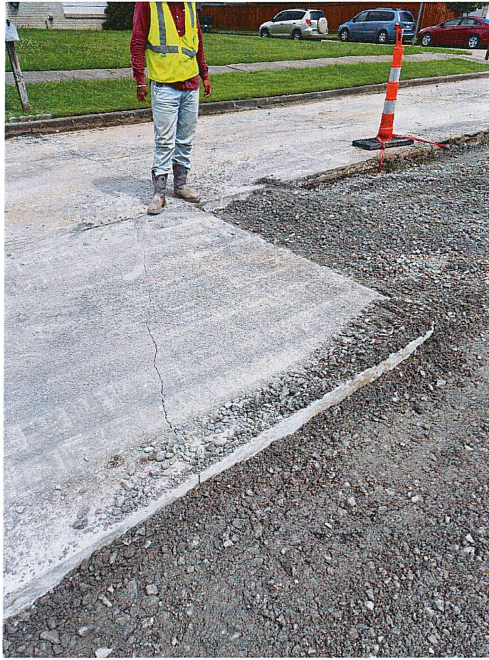
Figure 13: Structural crack from contractor rolling over slab
