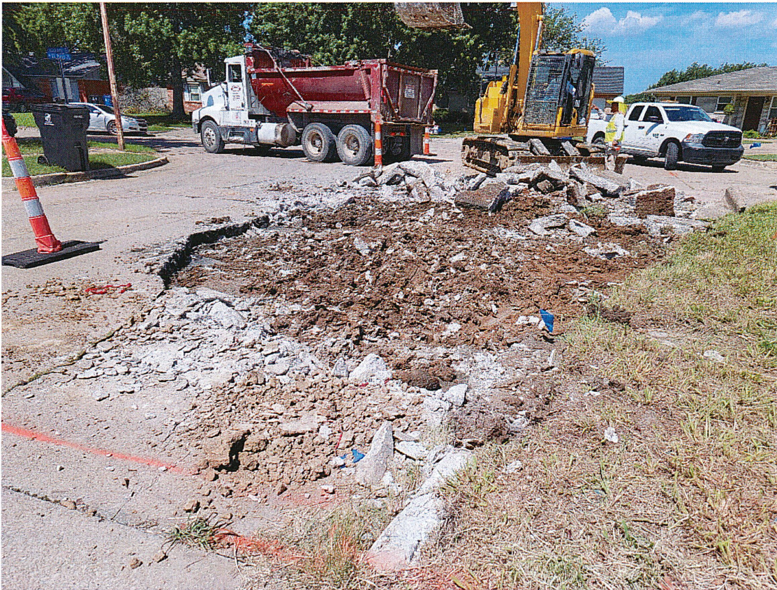
Figure 12: Active breaking using excavator
