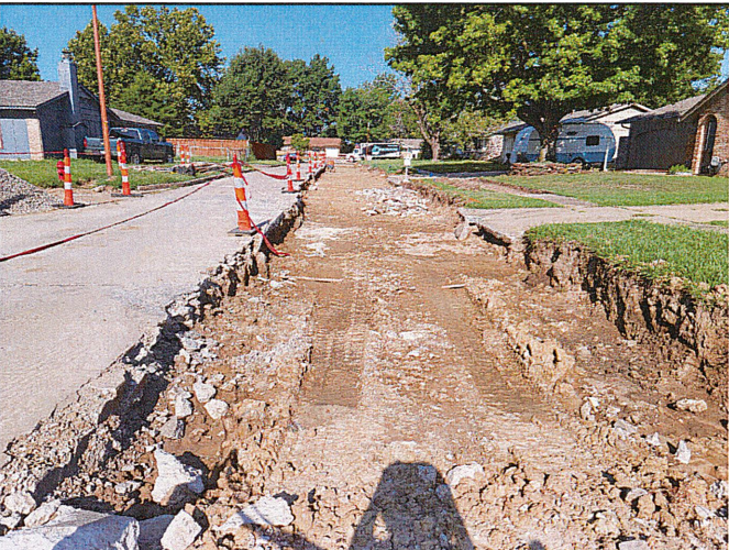
W. El Paso Pl. Dry solid subgrade. Holds up 4 ton skid loader.
