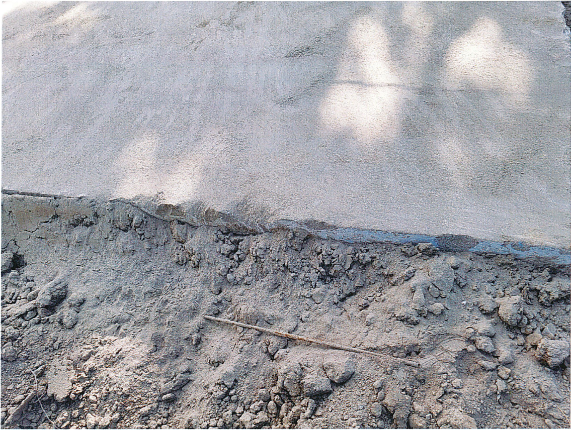
Figure 7: Chipping from excavator
