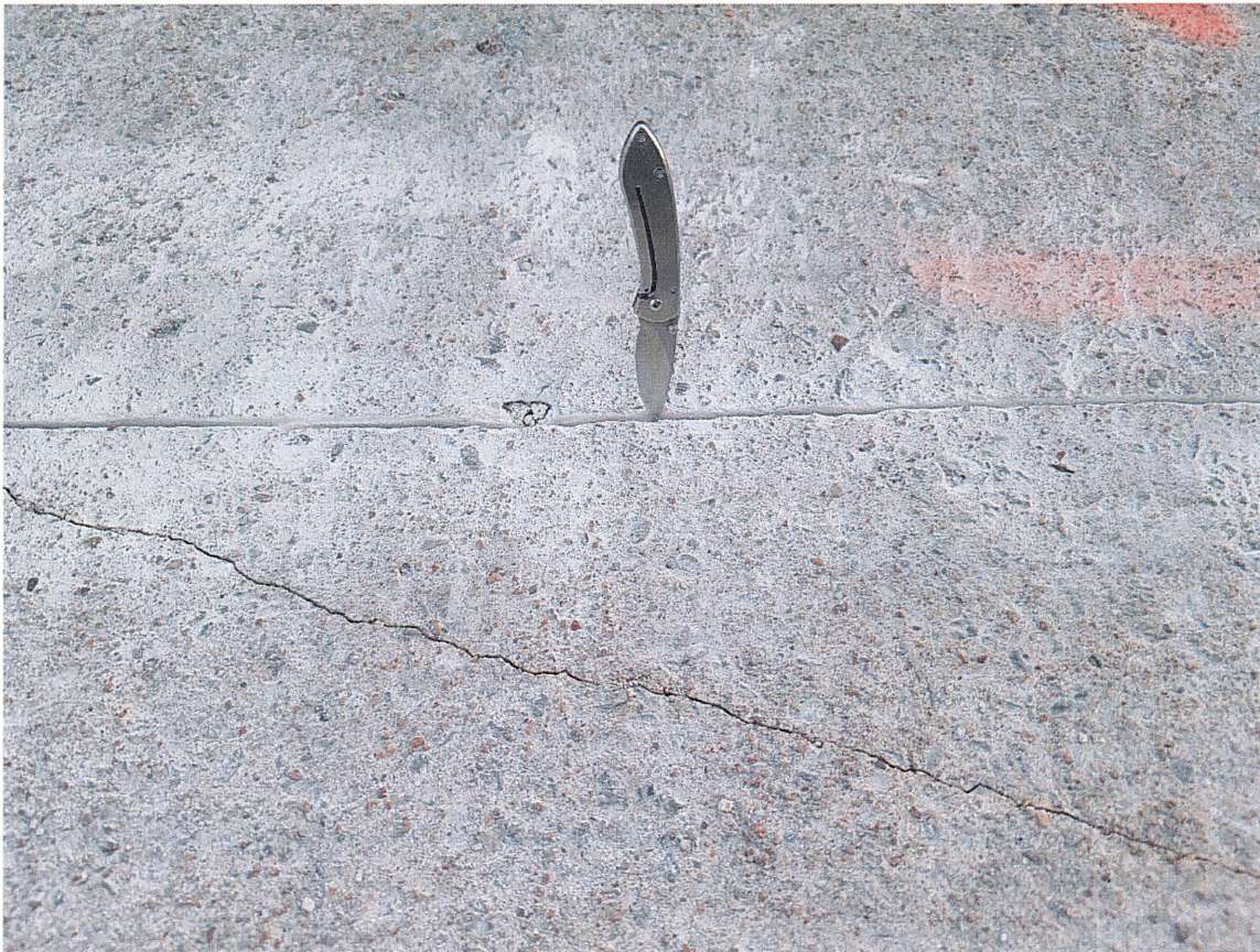
Figure 8: Improper sawcut depth
