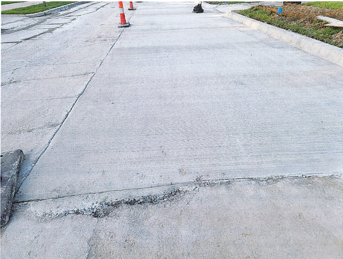
Figure 11: New edge cut due to chipping and improper methods
