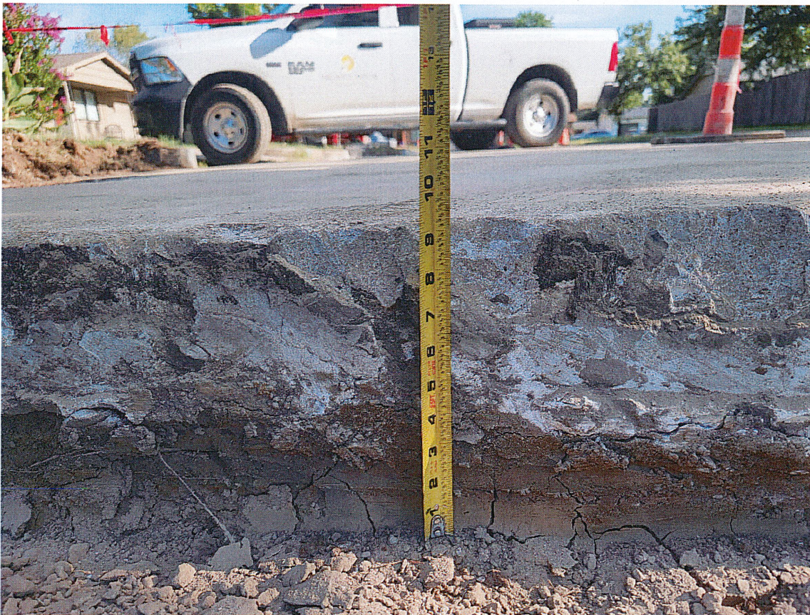
Figure 6: No saw cut and full depth concrete
