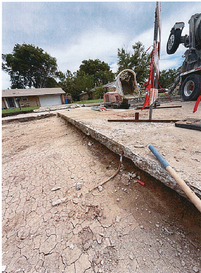
Figure 2: No Sawcut on right
