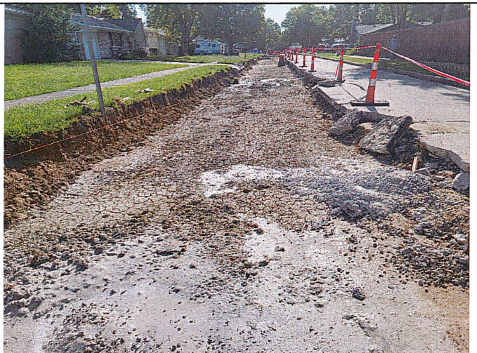
Subgrade is dry and solid. Contractor keeps letting the cement trucks wash out their trucks on to the subgrade.
