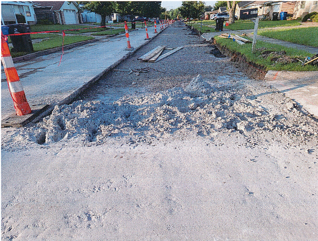
Figure 22: No Form Board on end of pour
