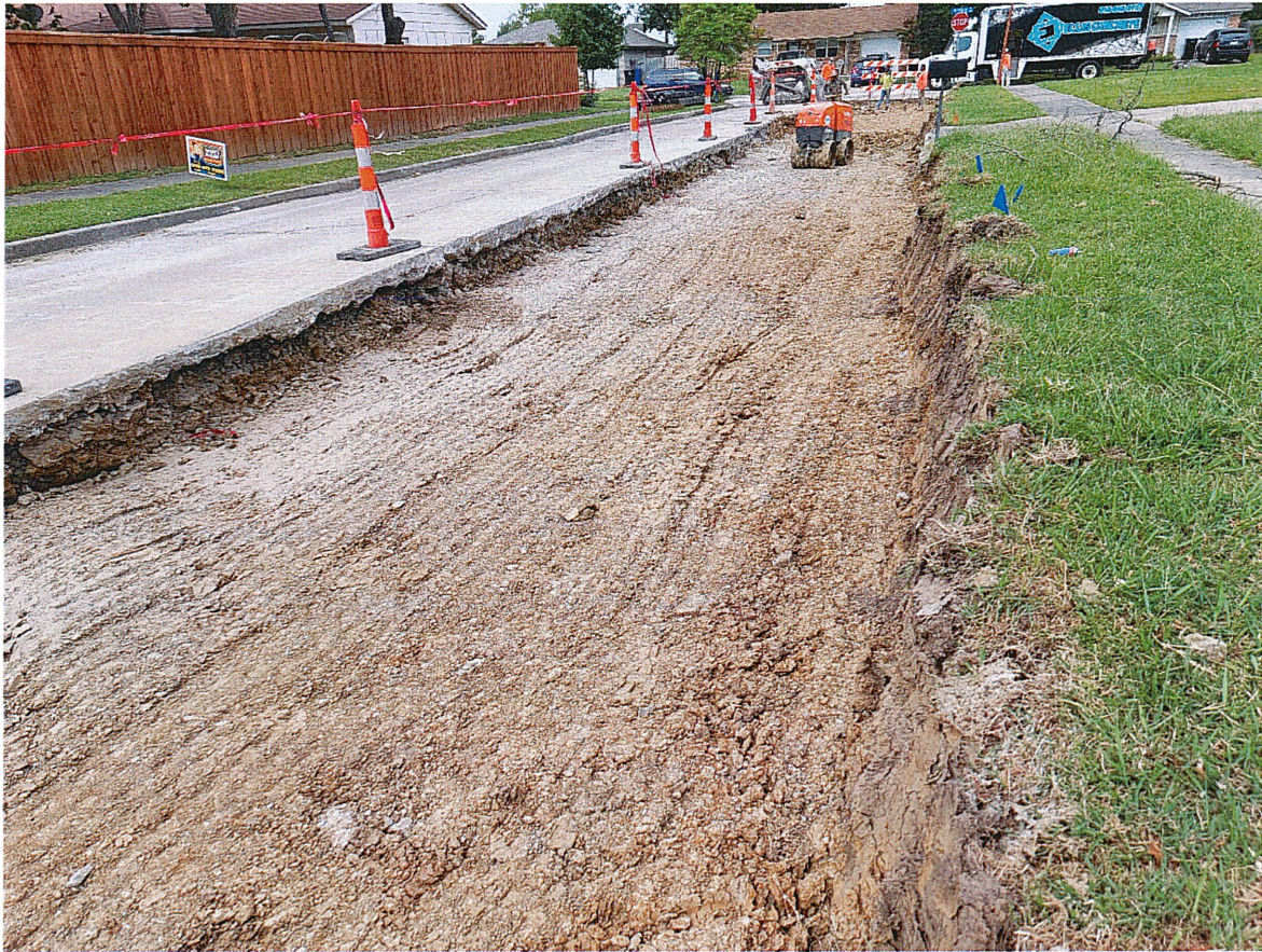
Figure 19: Contractor trying to compact when too wet
