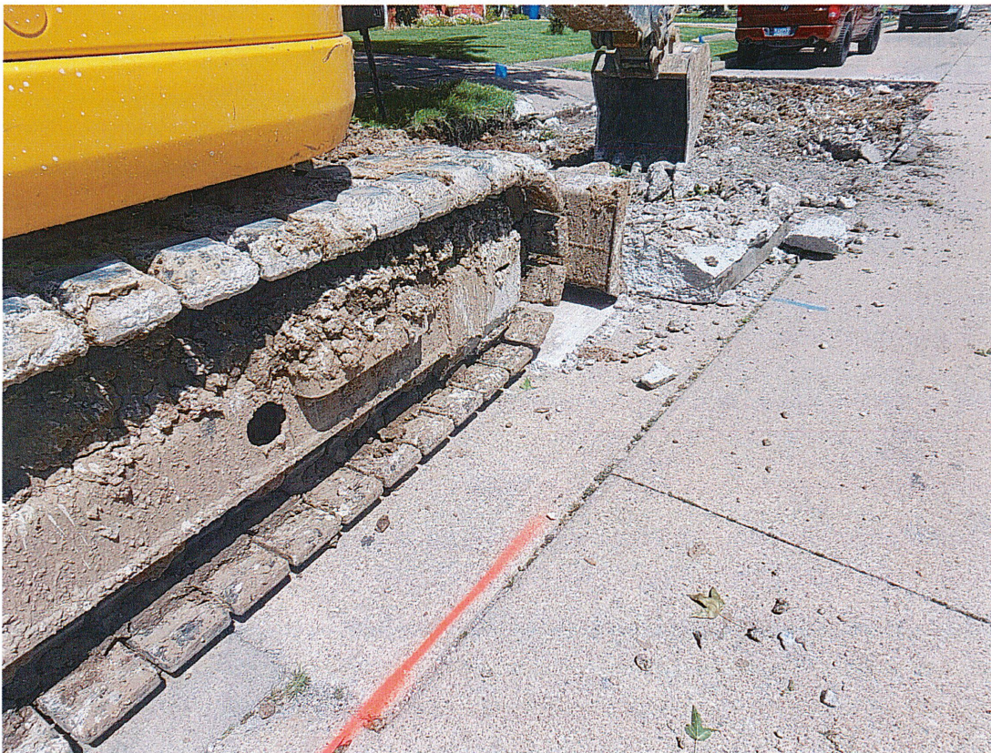
Figure 14: Showing active use of excavator to break
