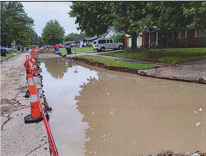
Subgrade holding 2' of water.
