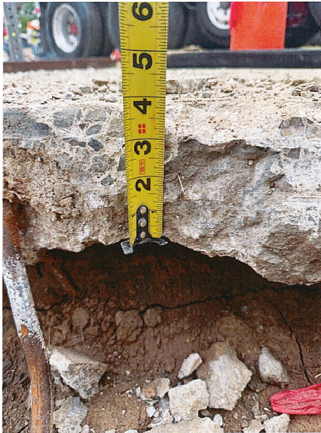
Figure 1: Underbreakage and dowel bent due to no sawcut
