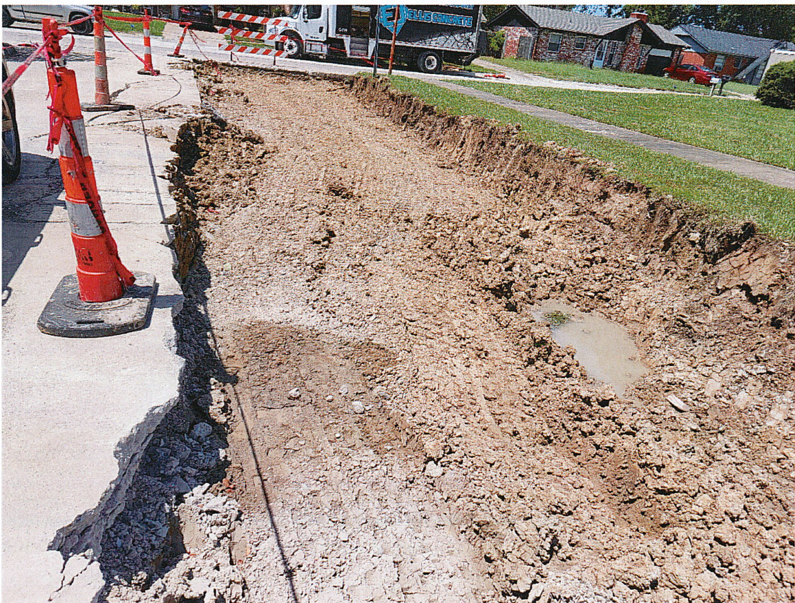
Figure 18: Failed roll test on subgrade
