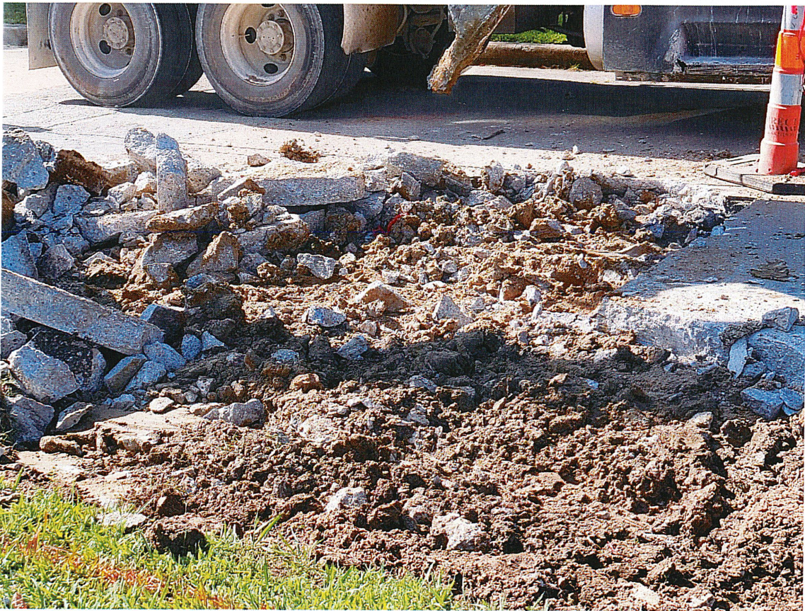
Figure 9: Upper Edge no saw cut, chipped, and underbreakage
