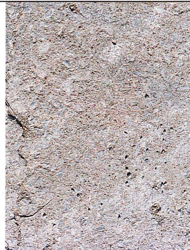
Subgrade is dry and solid. Contractor keeps letting the cement trucks wash out their trucks on to the subgrade.
