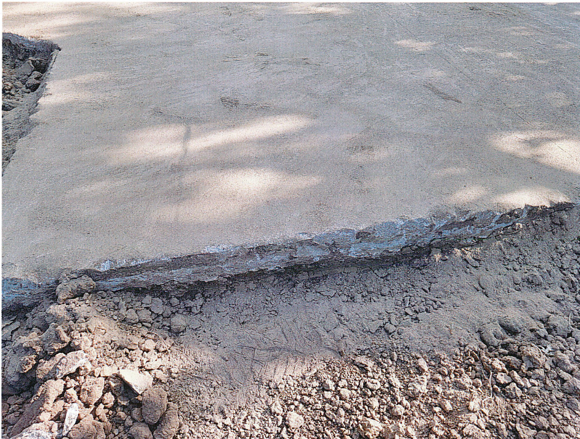
Figure 4: Chipping, scouring
