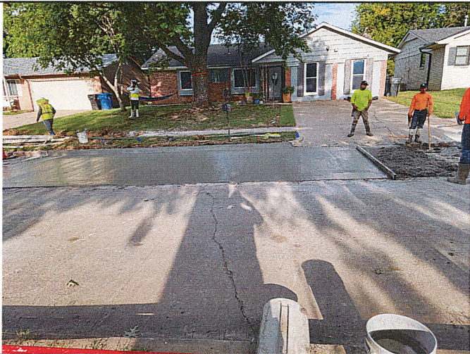
Waiting on next truck, unfinished concrete drying out Hickory Avenue
