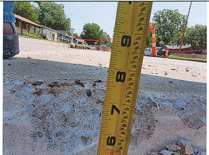
Existing concrete 7-3/4 inches thick El Paso Place
