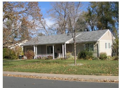
Figure 3.1 (top), Figure 3.2 (center) and Figure 3.3 (bottom) illustrate three styles of the Single-Family building form.
