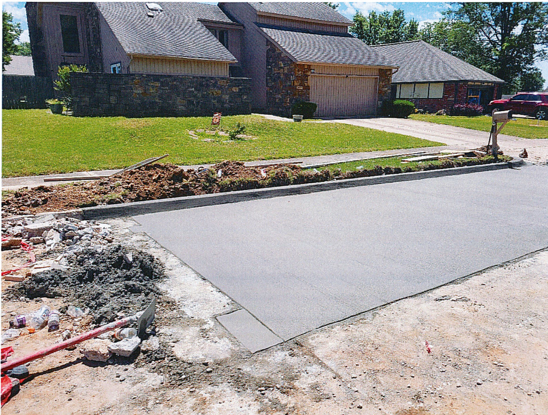
Figure 7: Improper edge line due to chipping
