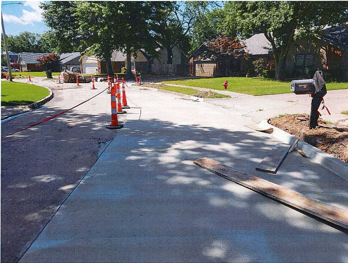
Figure 13: showing centerline being filled due to chipping
