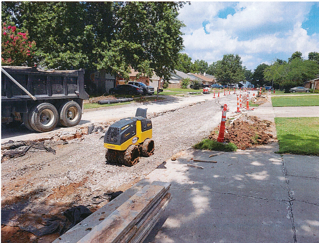
Figure 20: Showing material too wet to compact
