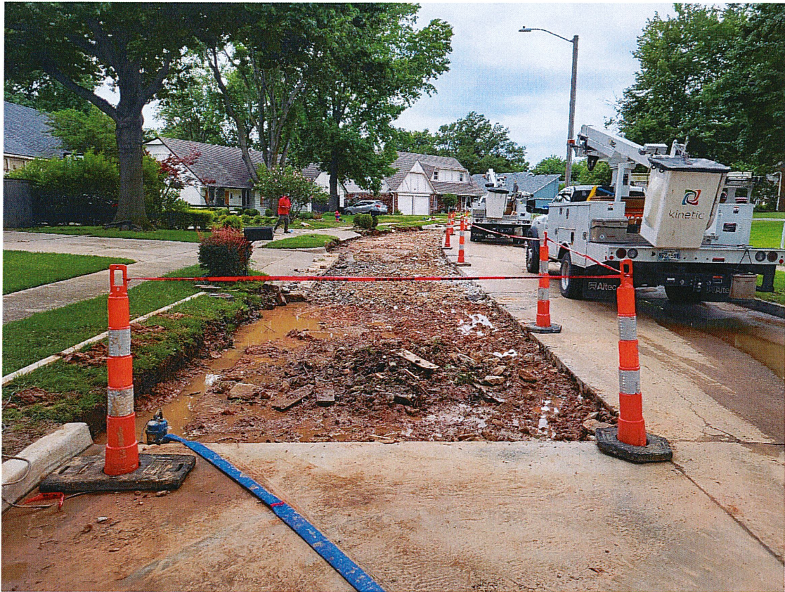
Figure 21: No excavation 1 foot past curb
