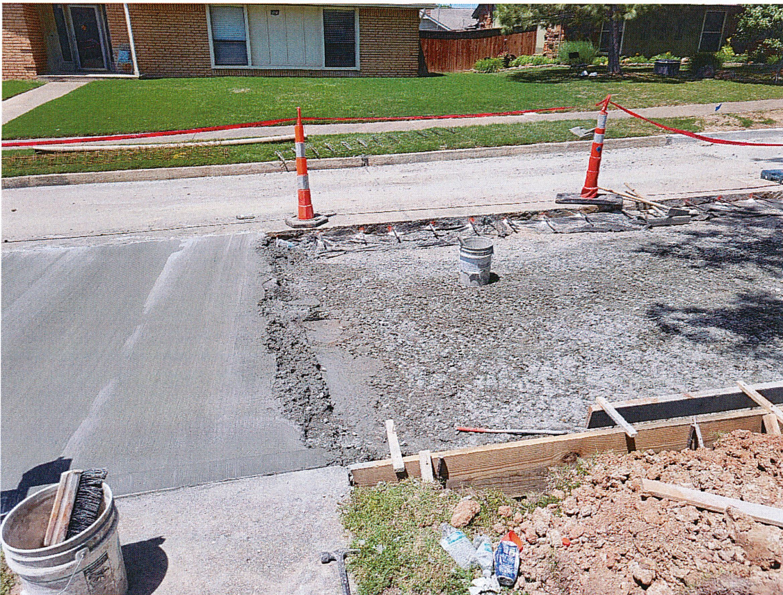
Figure 22: No Form Board on end of pour
