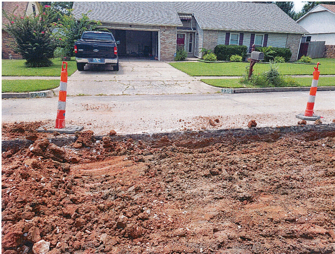
Figure 4: Subgrade too wet, chipping, scouring
