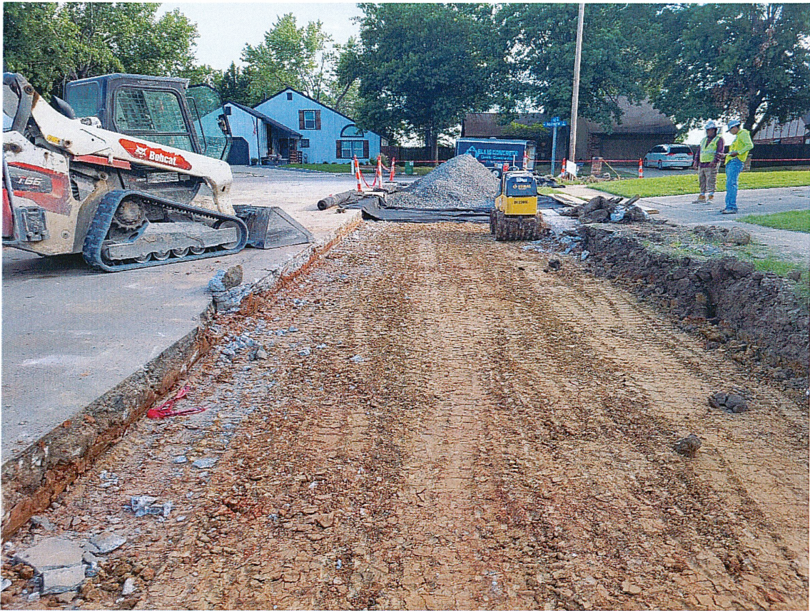
Figure 9: Left Edge scoured, chipped and underbreakage
