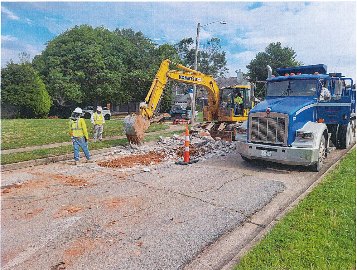
Figure 12: Active breaking using excavator
