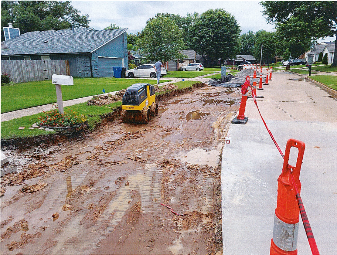
Figure 19: Contractor trying to compact when too wet
