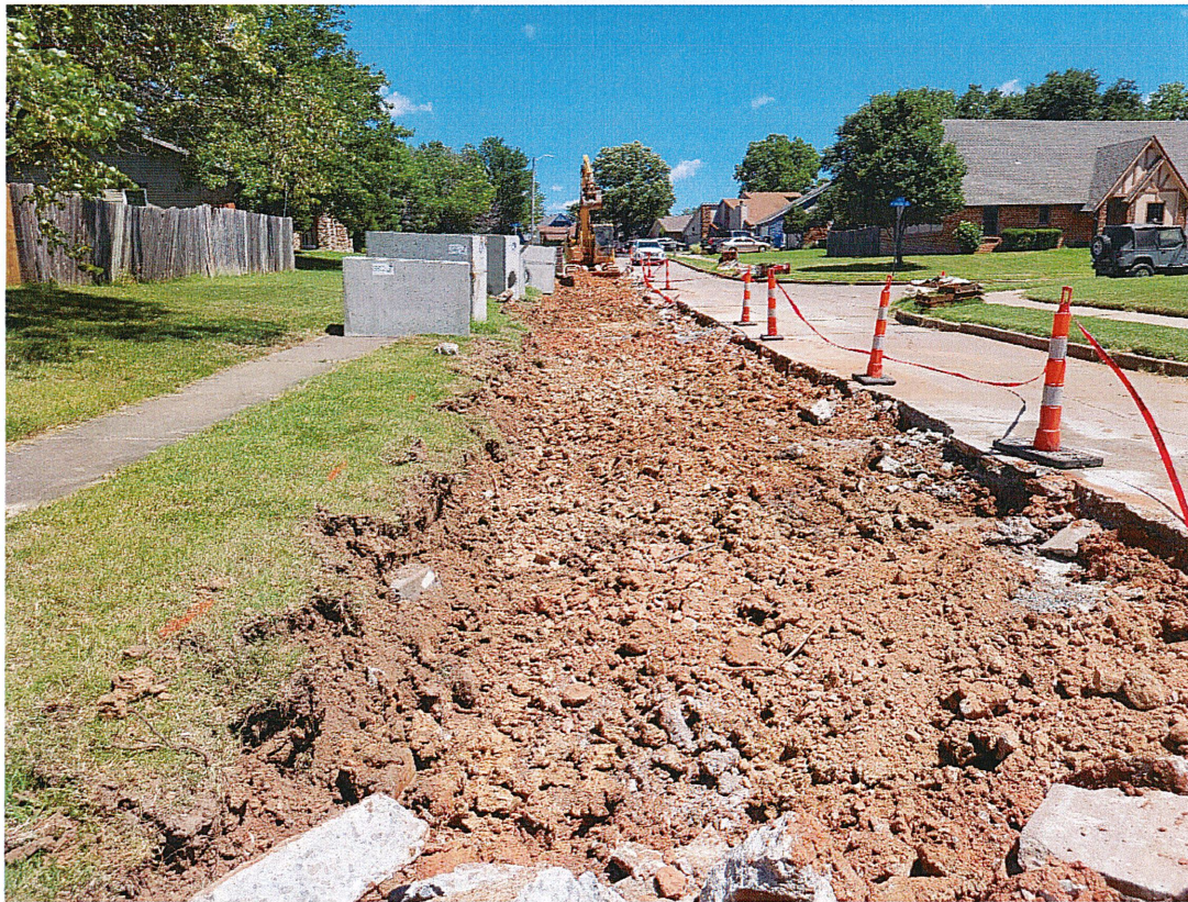
Figure 2: No Sawcut on right
