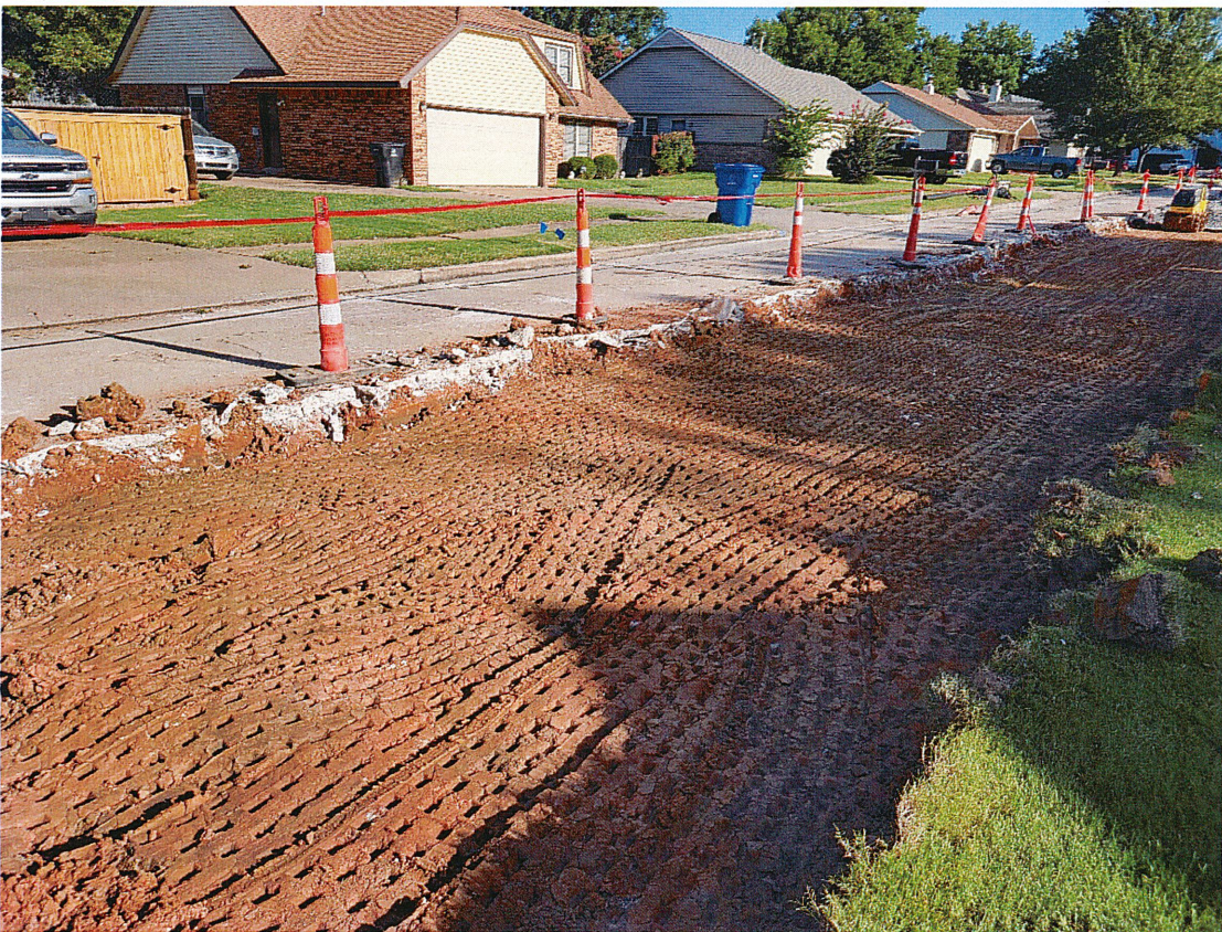
Figure 18: Failed roll test on subgrade
