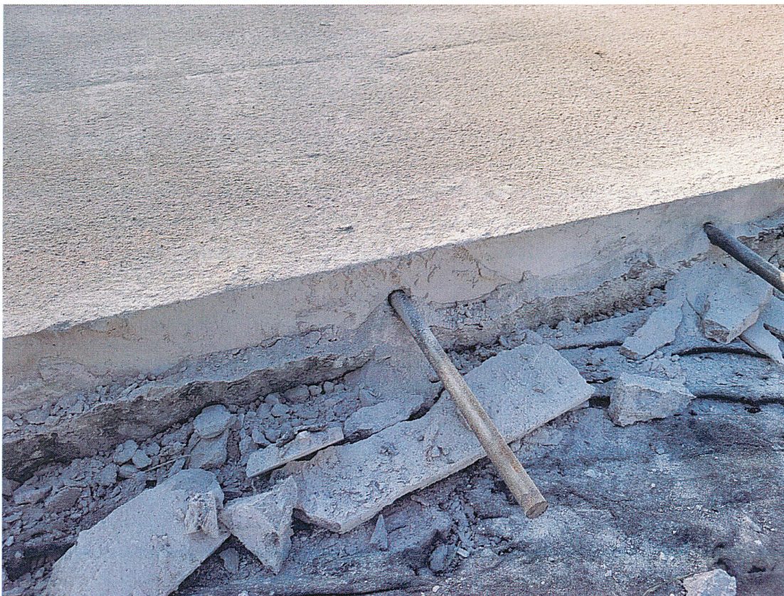
Figure 8: no epoxy, improper sawcut depth
