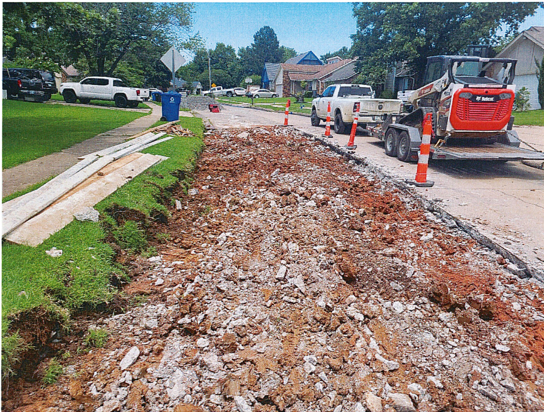
Figure 3: Scouring on right but not full depth cut, dowels still intact from no sawcut
