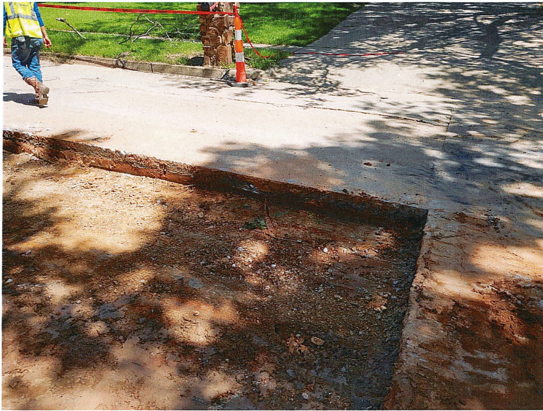
Figure 1: Improper Depth of Sawcut
