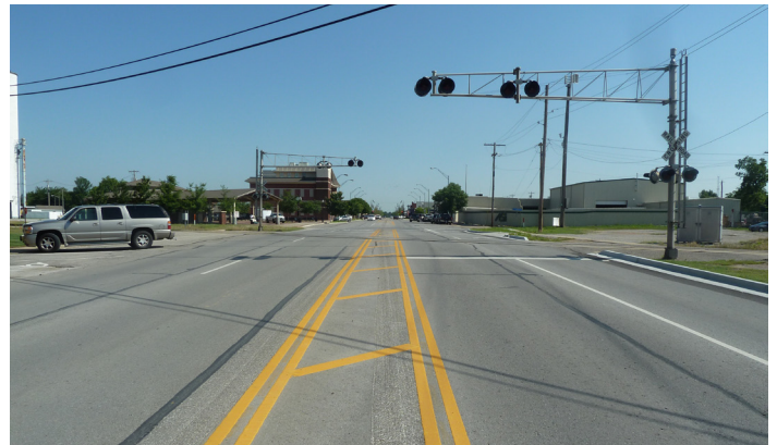
Typical crosswalk on West Main Street
