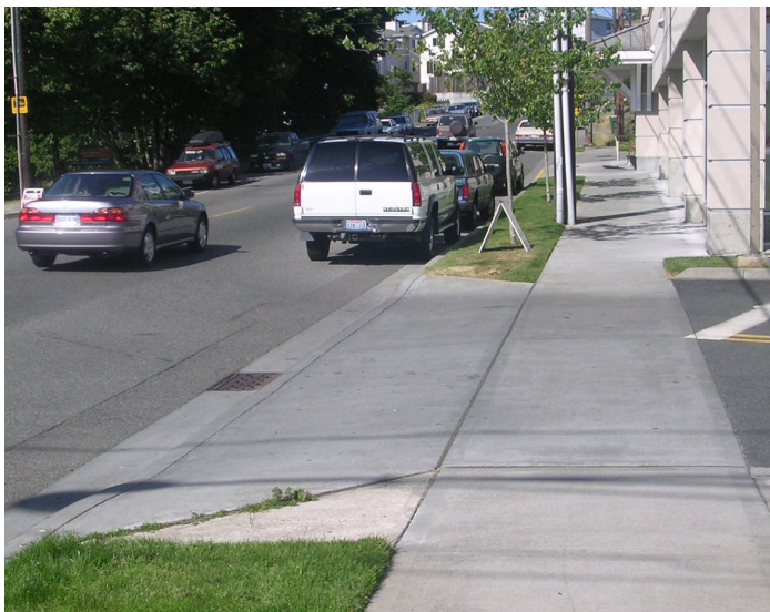
Sidewalk Crossing Driveway
