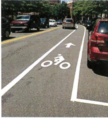
BIKE LANES ARE MARKED WITH A BICYCLIST SYMBOL AND ARROW INDICATING DIRECTION OF TRAVEL
