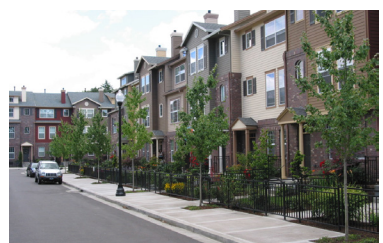
Figure 3.10 (top) and Figure 3.11 (bottom) illustrate the Rowhouse building form that shows street-facing entries and distinguishes between each rowhouse unit through the use of wall offsets and changes in material.
