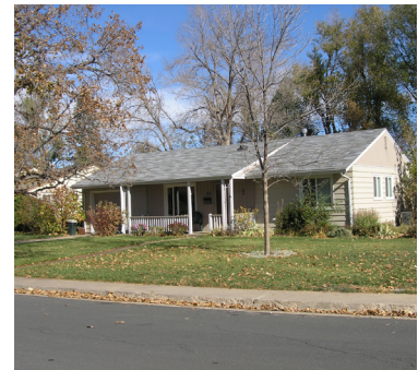
Figure 3.3 Illustrates the Single-Family B building form is one-story in height and is horizontally aligned to the street.
